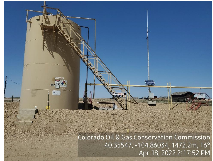
Photo 4: Centralized Tank Battery
