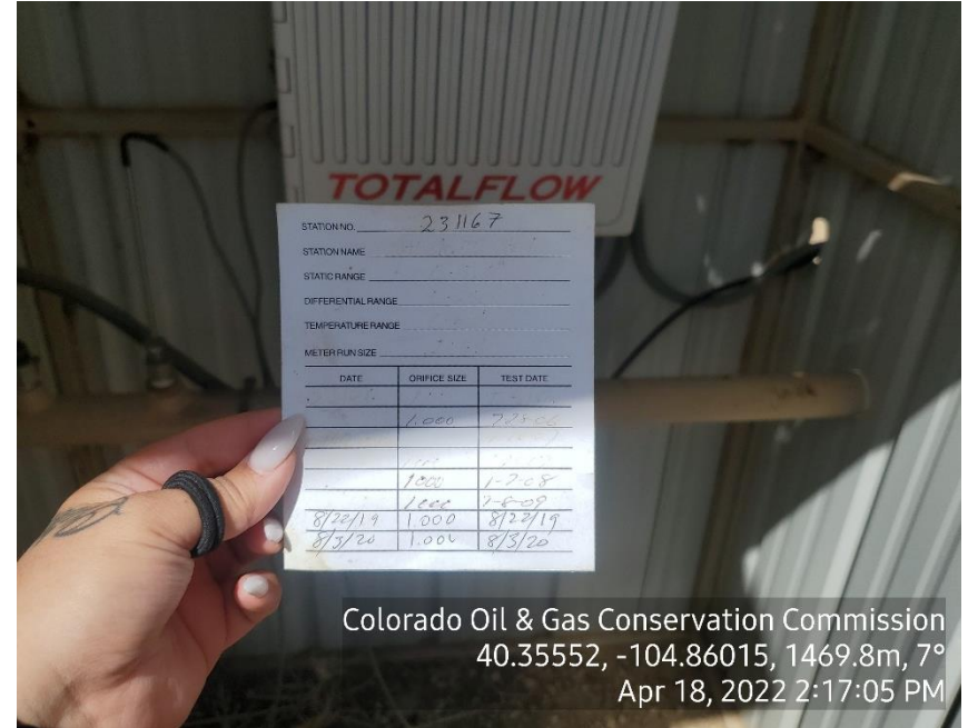
Photo 6: Gas meter not annually calibrated
