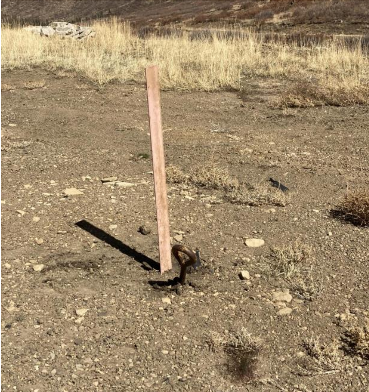
PHOTO 2: THE ANCHOR MARKER WAS INSTALLED ON ANCHOR. CORRECTIVE ACTION COMPLETED ON 4/19/2022.
