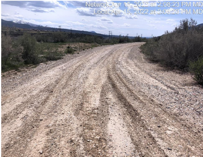
Photo #6464 Insufficient tracking BMP at entrance to location.
