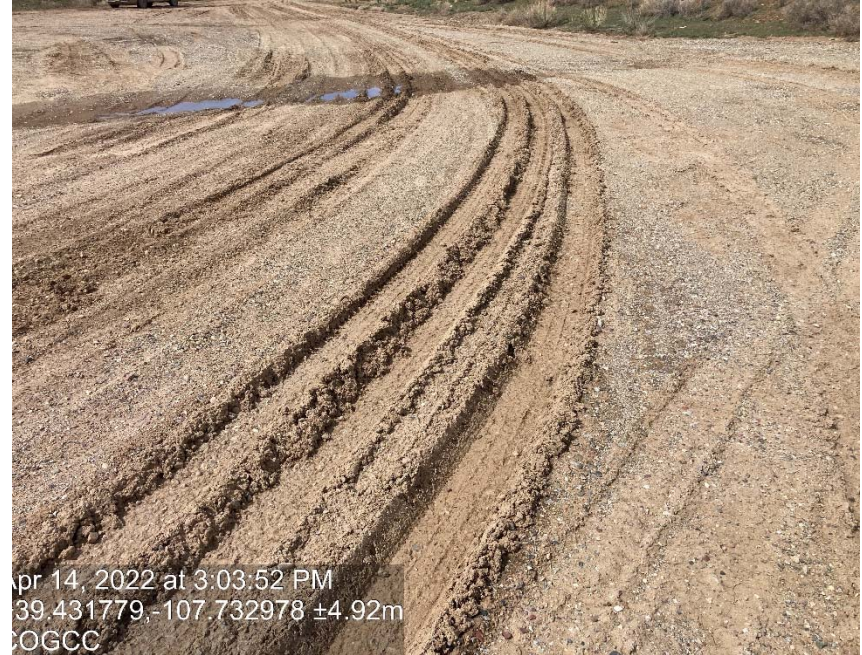
Lack of stabilization/compaction
