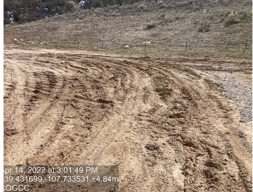
Lack of stabilization/compaction
