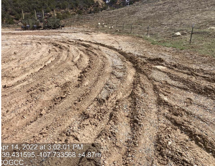
Lack of stabilization/compaction
