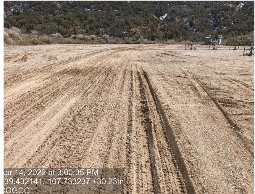
Lack of stabilization/compaction
