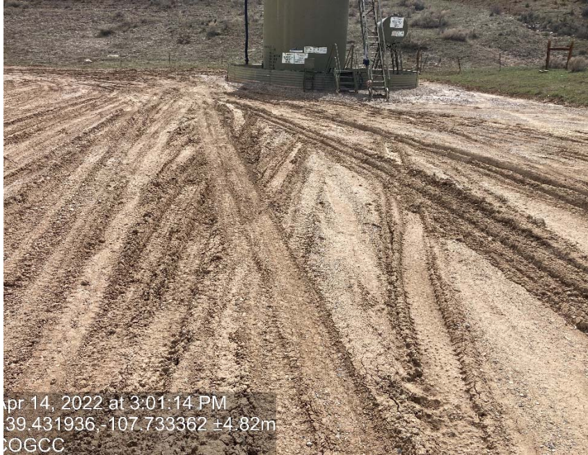
Lack of stabilization/compaction
