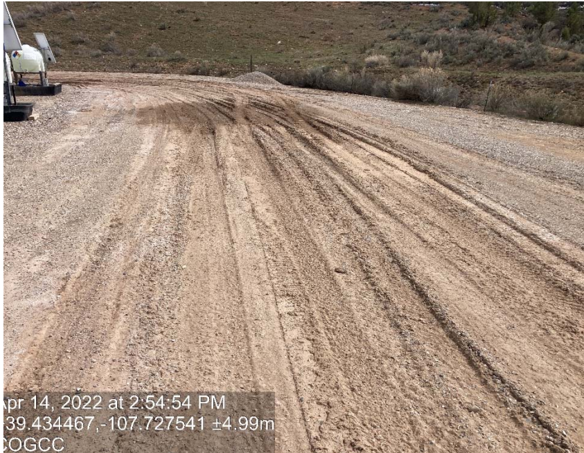
Lack of stabilization/compaction
