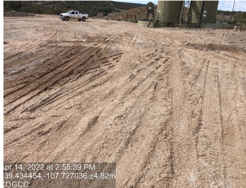
Lack of stabilization/compaction
