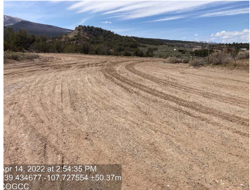
Lack of stabilization/compaction
