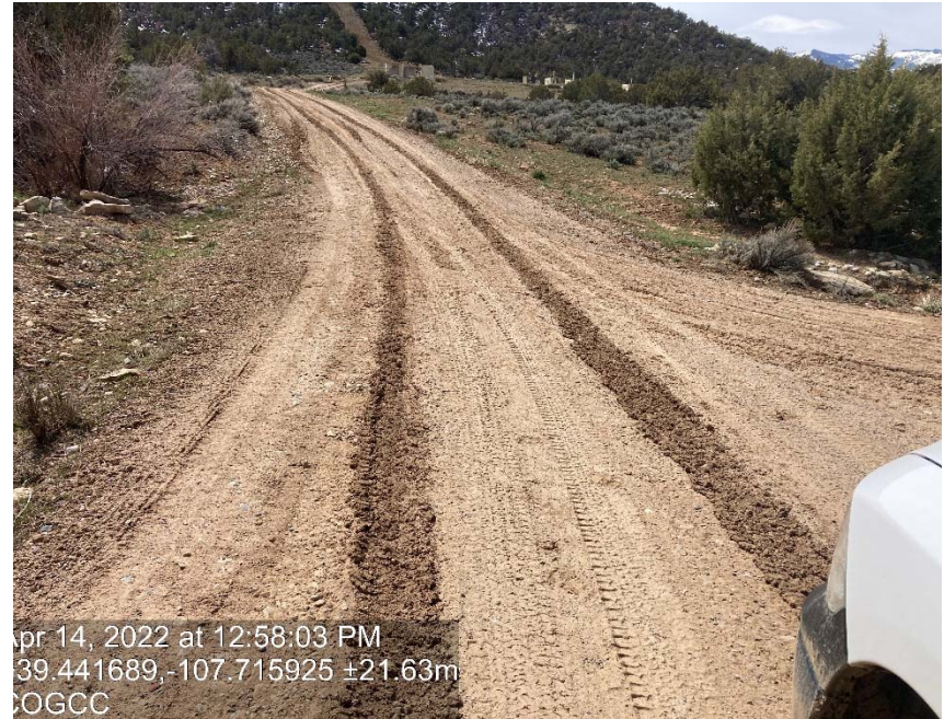
Lack of stabilization/compaction
