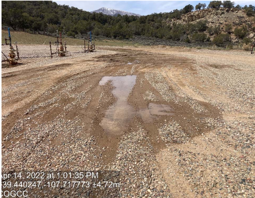
Lack of stabilization/compaction
