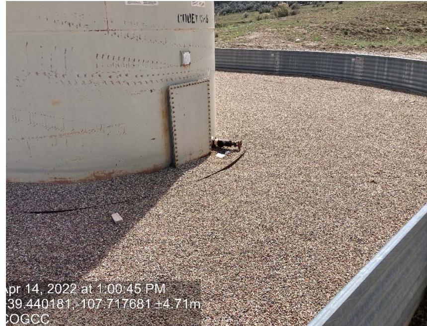
Valve missing cap/plug
