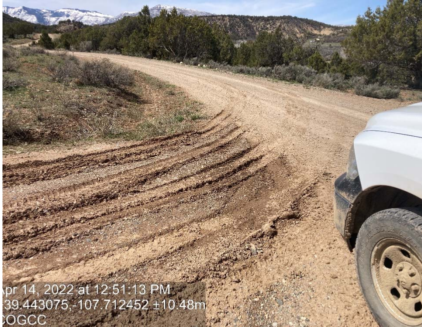
Lack of stabilization/compaction
