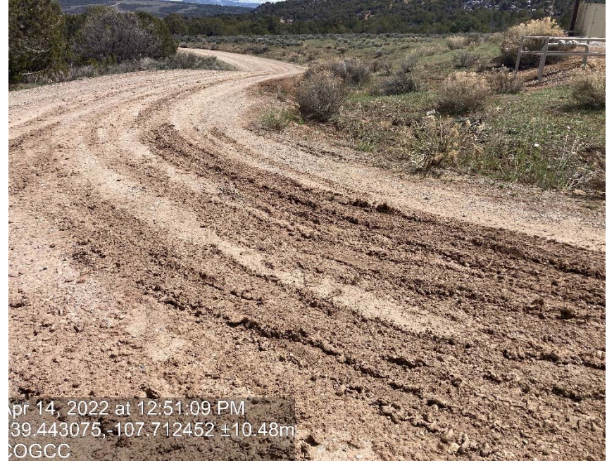
Lack of stabilization/compaction
