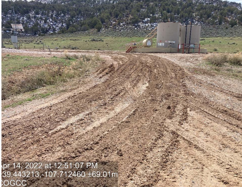
Lack of stabilization/compaction
