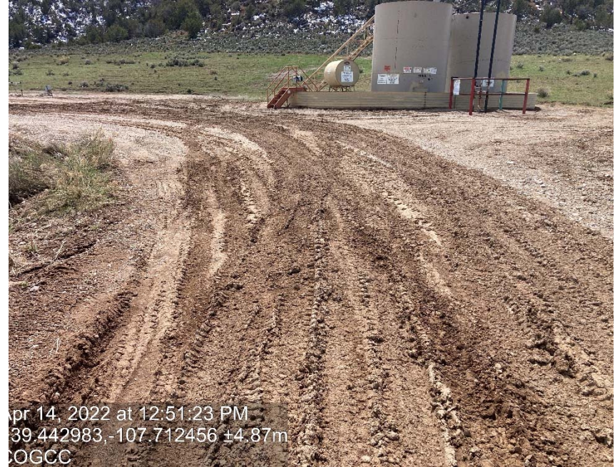
Lack of stabilization/compaction
