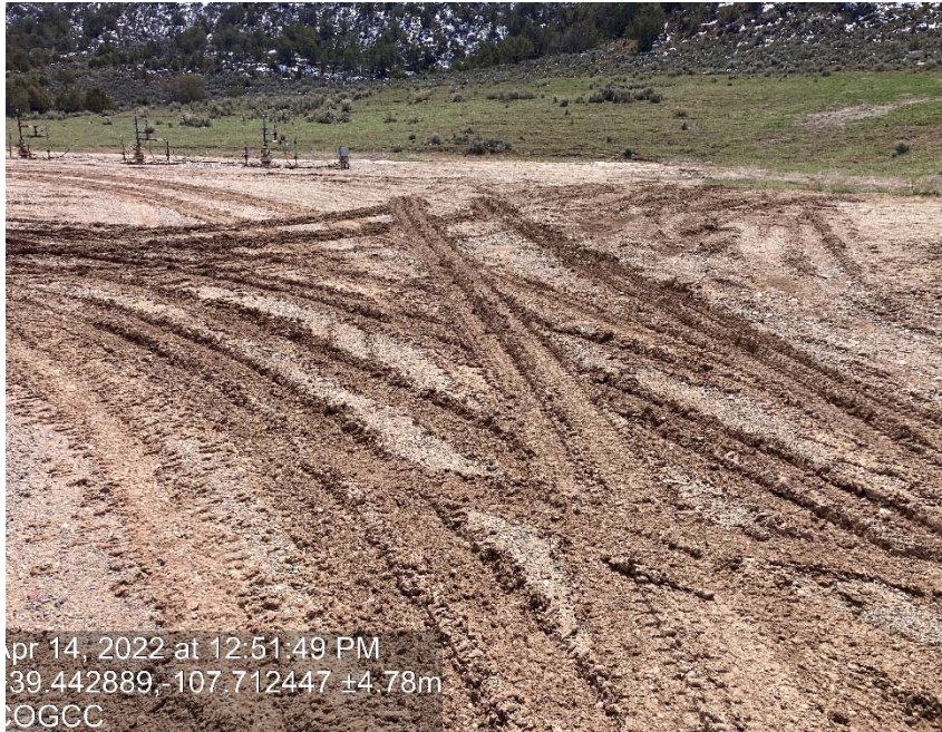
Lack of stabilization/compaction
