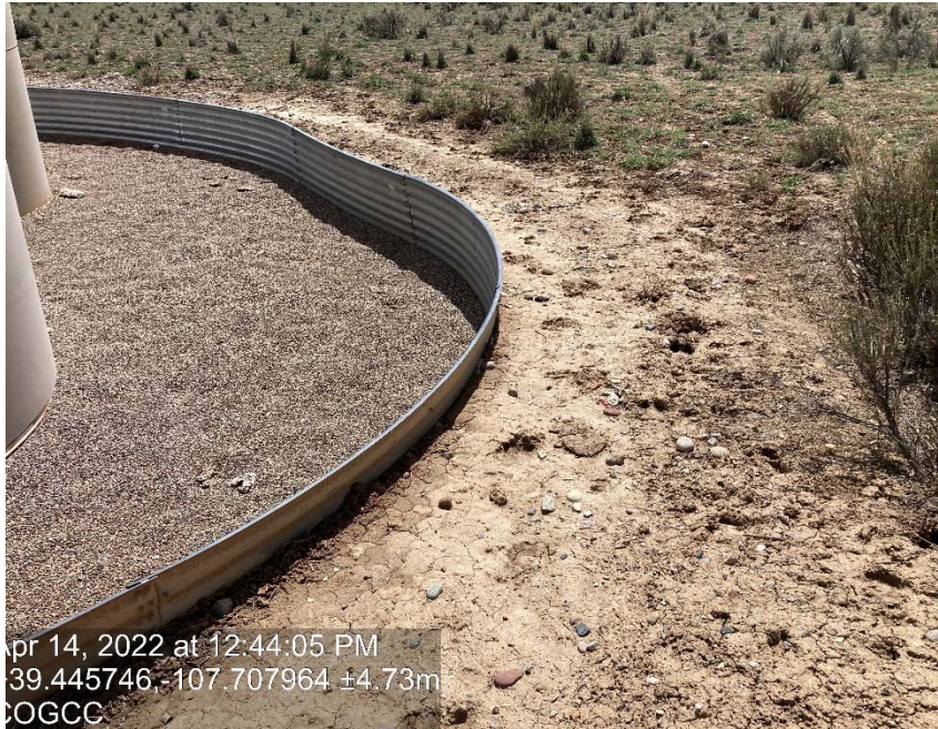
Sediment piled up on battery containment
