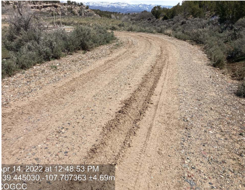
Lack of stabilization/compaction
