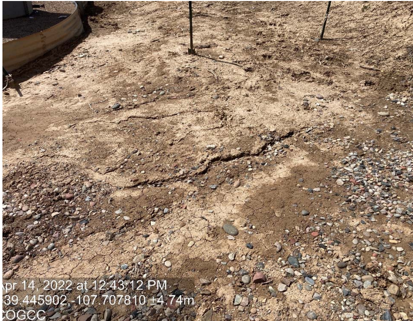
Lack of stabilization/ compaction/ erosion
