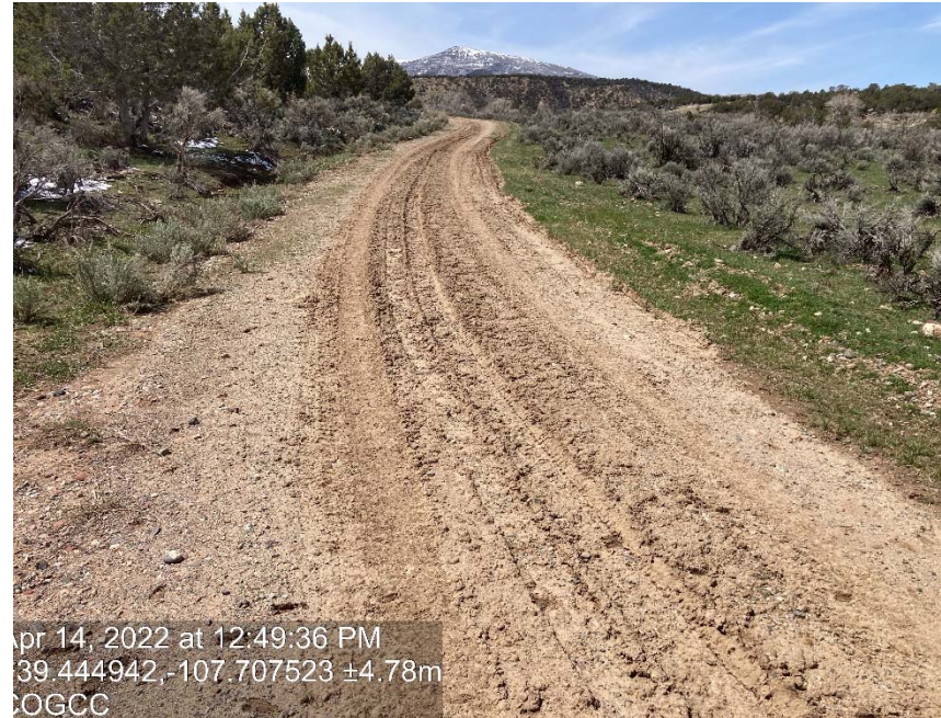
Lack of stabilization/compaction
