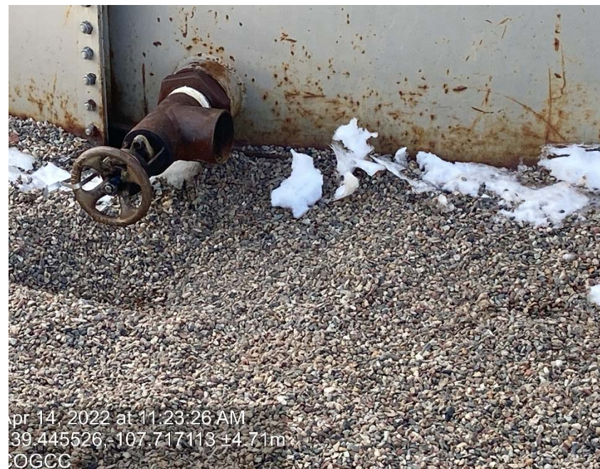
Valve missing cap/plug
