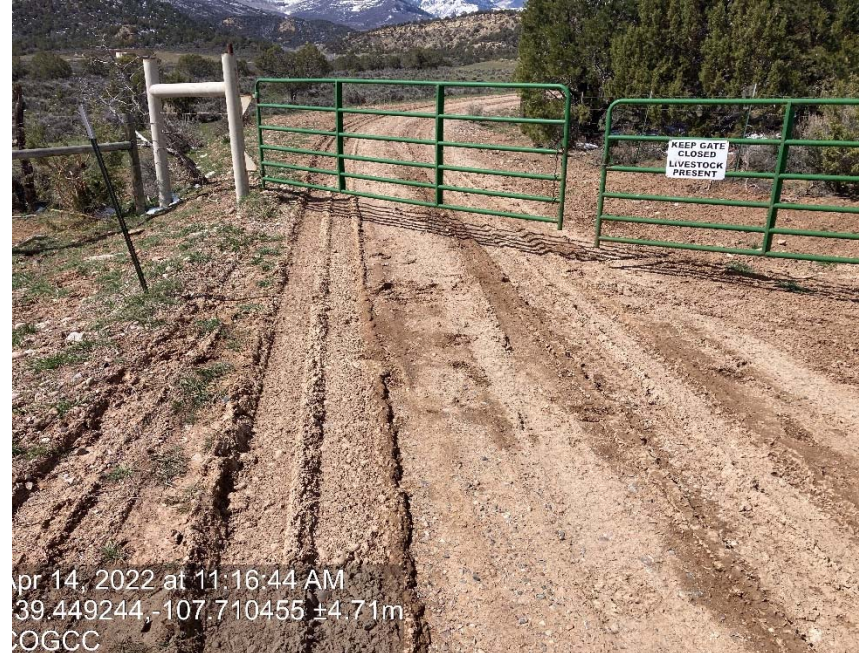
Lack of stabilization/compaction
