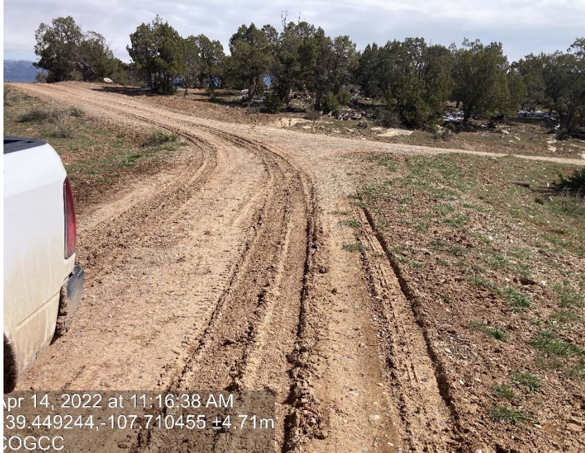
Lack of stabilization/compaction
