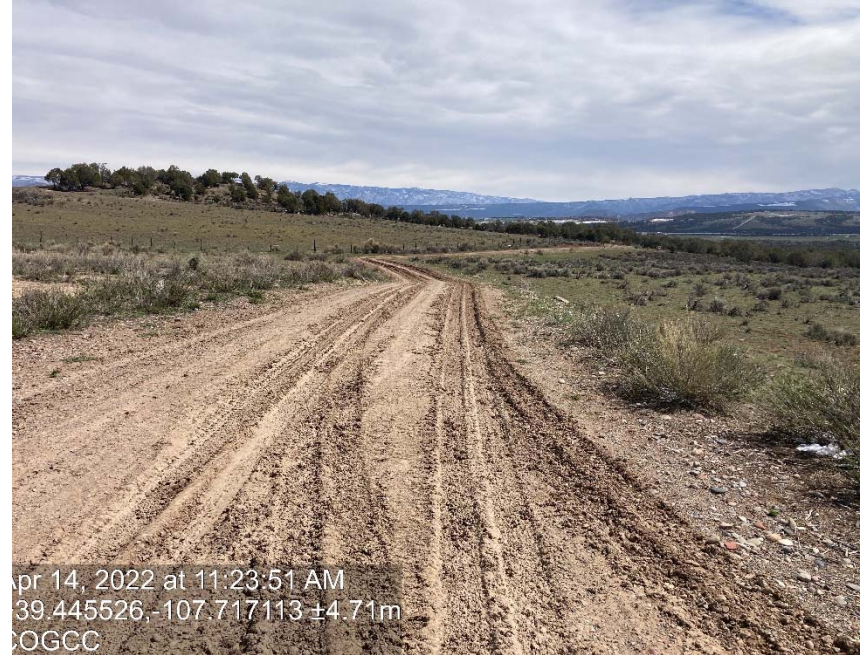
Lack of stabilization/compaction
