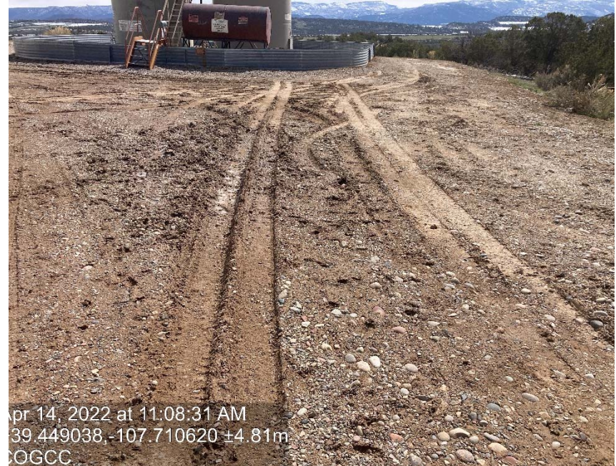
Lack of stabilization/compaction
