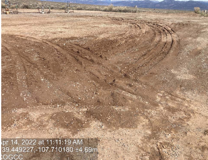
Lack of stabilization/compaction
