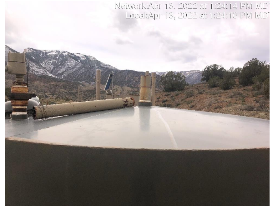
Photo #6431 Vent pipe on tank open ended.
