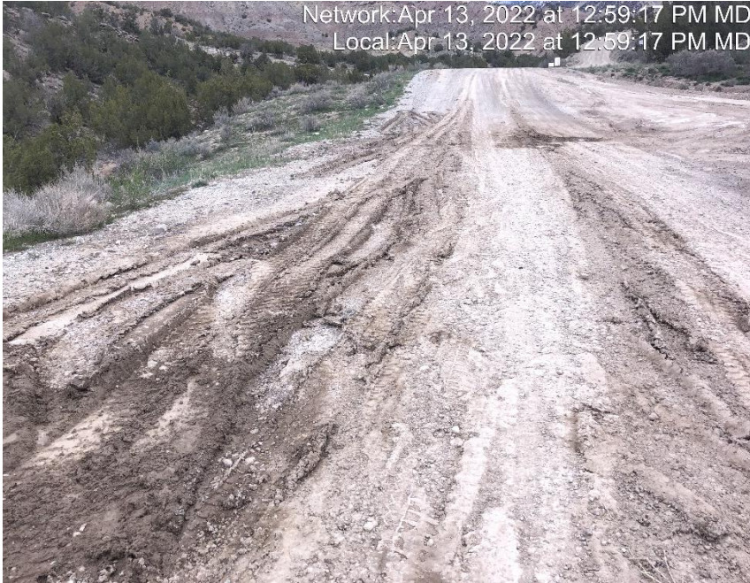
Photo #6427 Insufficient tracking BMP located at the entrance to location.
