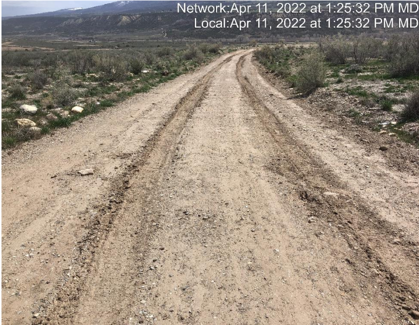
Photo #6412 Insufficient tracking BMP at entrance to location.
