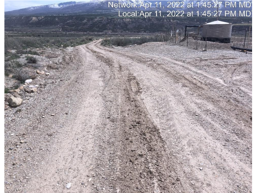
Photo #6416 Location lacks stabilization.
