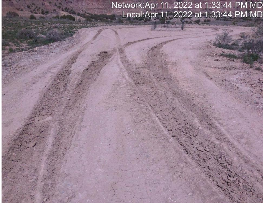
Photo #6415 Location lacks stabilization.
