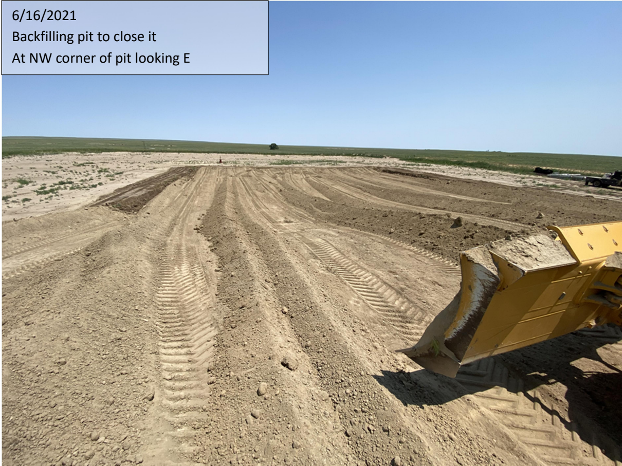
6/16/2021 Backfilling pit to close it At NE corner of pit looking W
