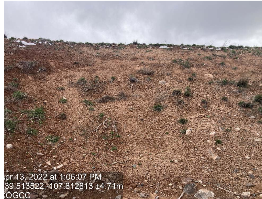
Lack of stabilization/ erosion
