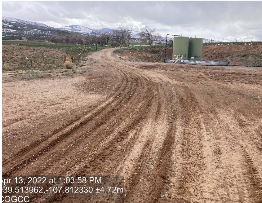
Lack of stabilization/ compaction/ degradation
