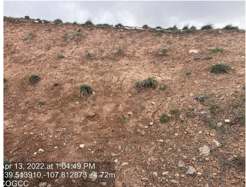
Lack of stabilization/ erosion
