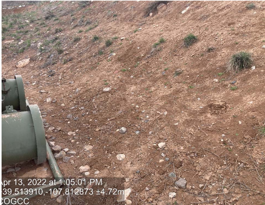
Lack of stabilization/ erosion
