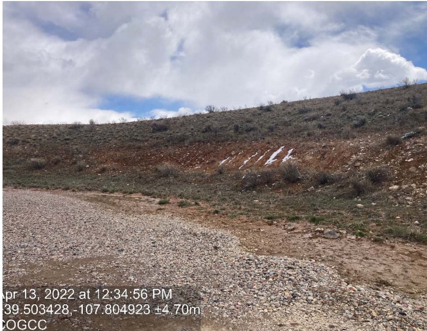
Cut slope shows signs of lack of stabilization/ erosion
