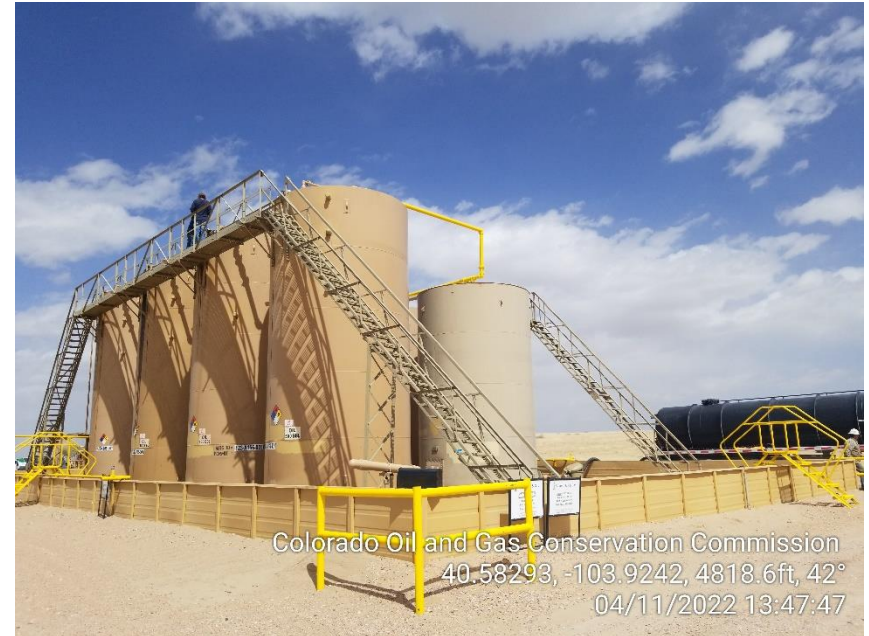
Photo 8 – Tank Battery – Oil Tanks
