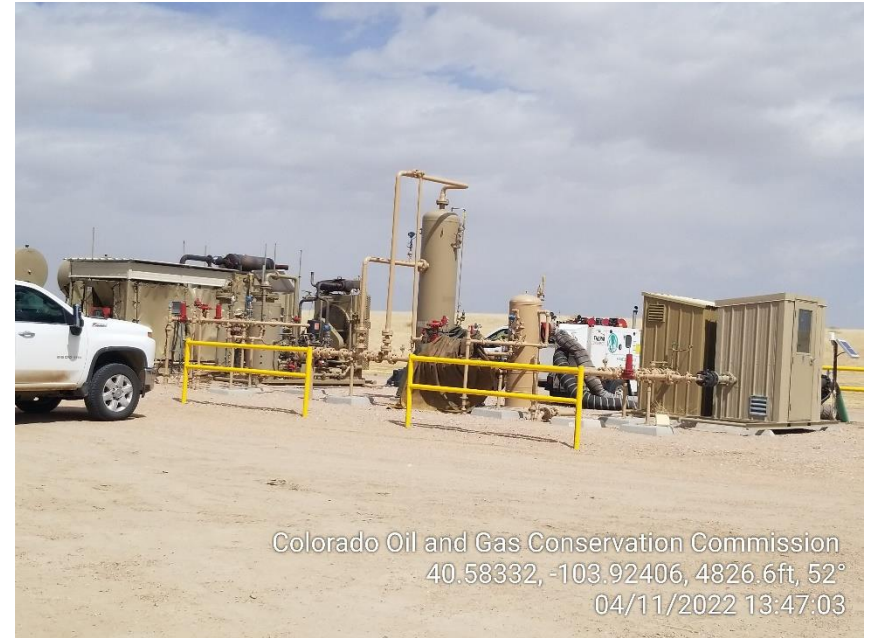
Photo 6 – Compressor, VRU and Gas Meters
