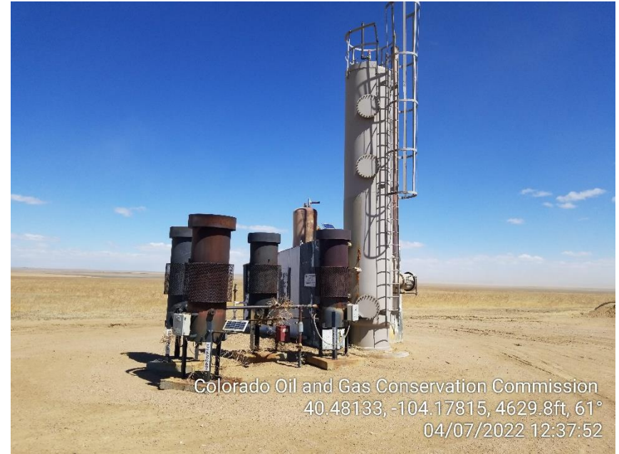
Photo 4 – Heater Treater and ECDs
