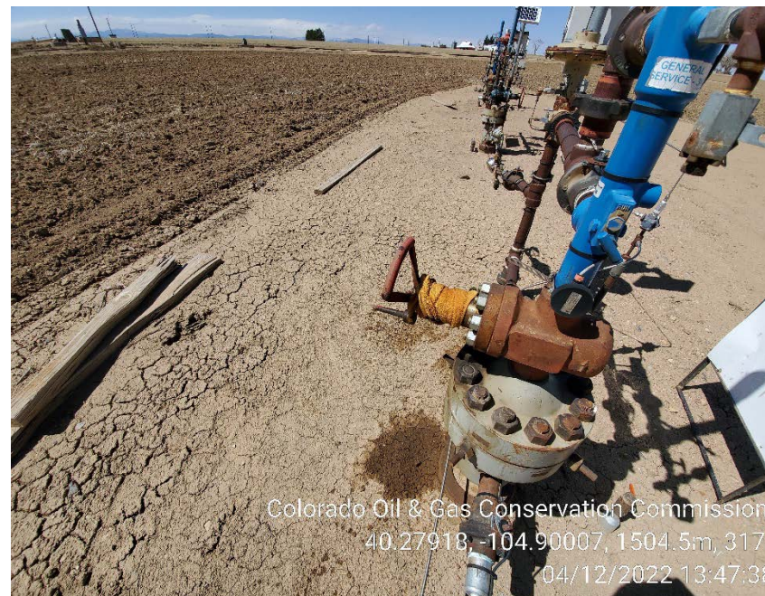
Master valve leak and stained soil
