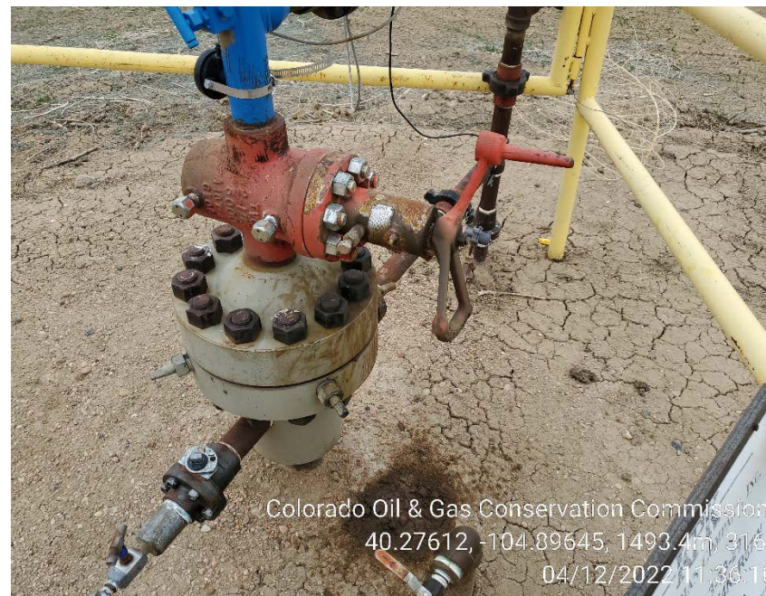
Master valve leak and stained soil
