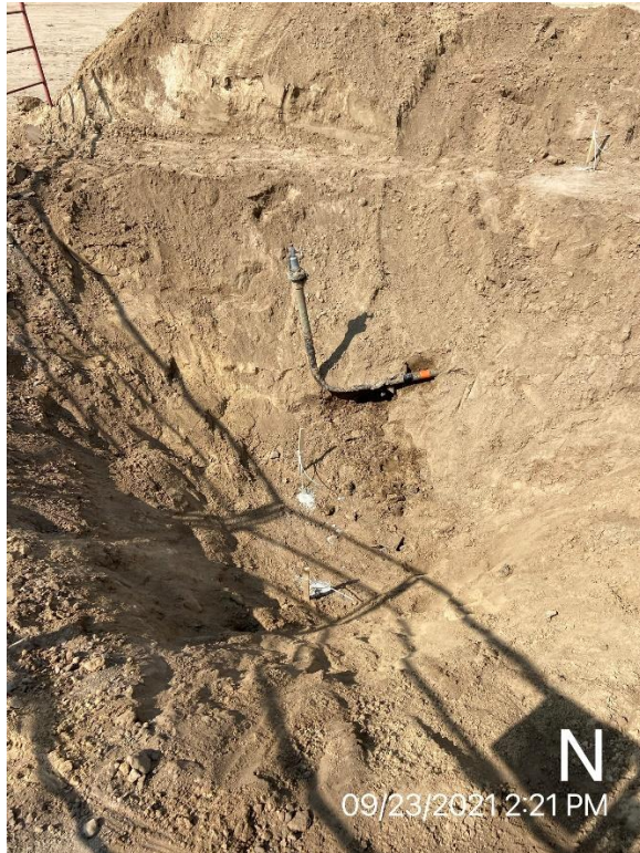
Ale W 29-21 Wellhead Excavation
