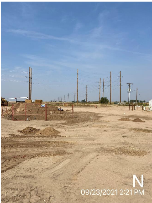
Ale W 29-21 Wellhead Excavation – Wide View
