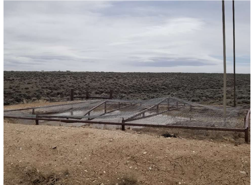
Photo 6. 2 of 2 pits. This pit does not have 2 feet of freeboard.
