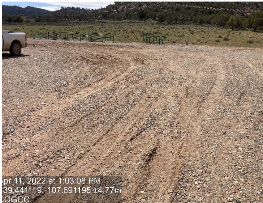
Some areas of lack of stabilization/compaction
