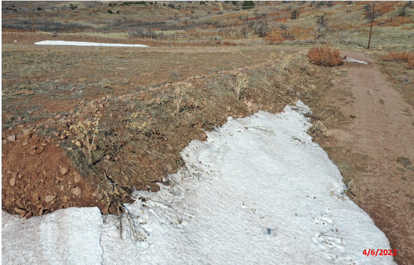
Photo 6. Facing northwest along the fill slope. There are numerous noxious weeds still remain along the fill slope. Noxious weeds observed include: Common mullien, Musk thistle, Plumeless thistle, and Scotch thistle.
