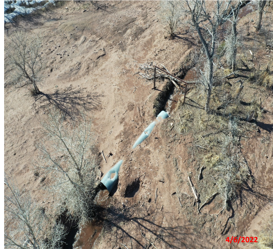
Photo 3. The culvert has become exposed due to erosion and is susceptible to further erosion and potential washout.
