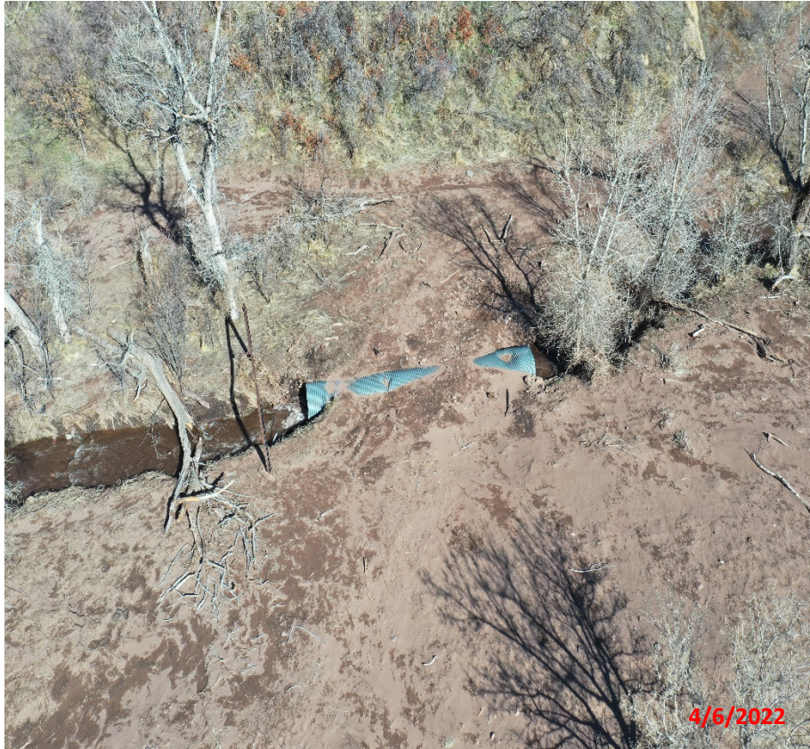
Photo 2. Drone aerial photo facing toward the access road which crossing the perennial stream. The culvert has become exposed due to erosion and is susceptible to further erosion.
