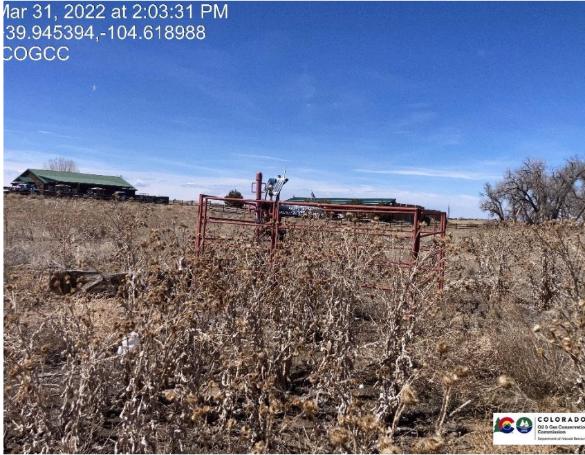
Pic 1 wellhead. Wellhead is located inside Colorado Clays shooting range
