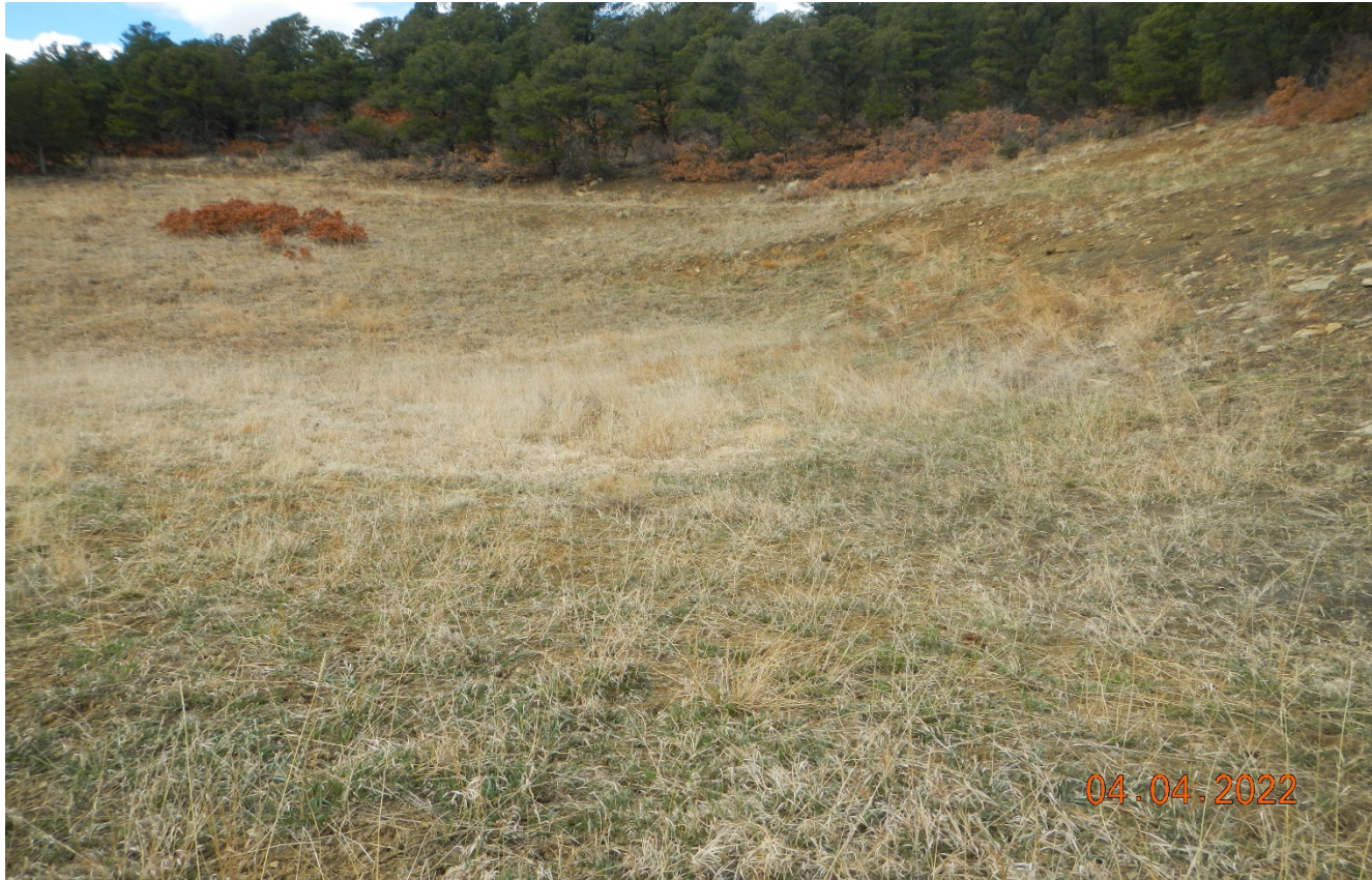
Photo 6. Facing toward the cut slope which is stabilized with perennial vegetation.
