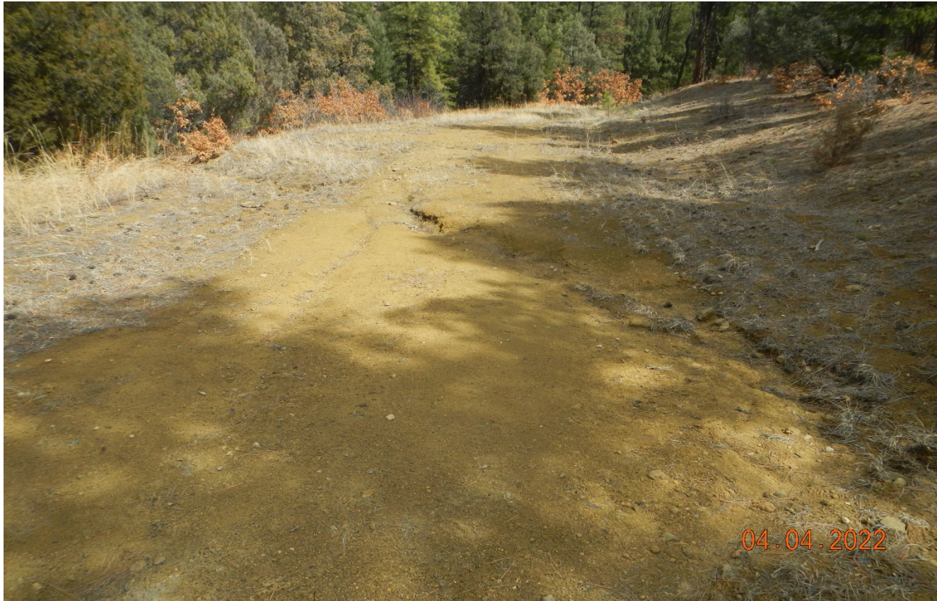
Photo 2. There is signs that stormwater has eroded over the water bar shown at red arrow.
