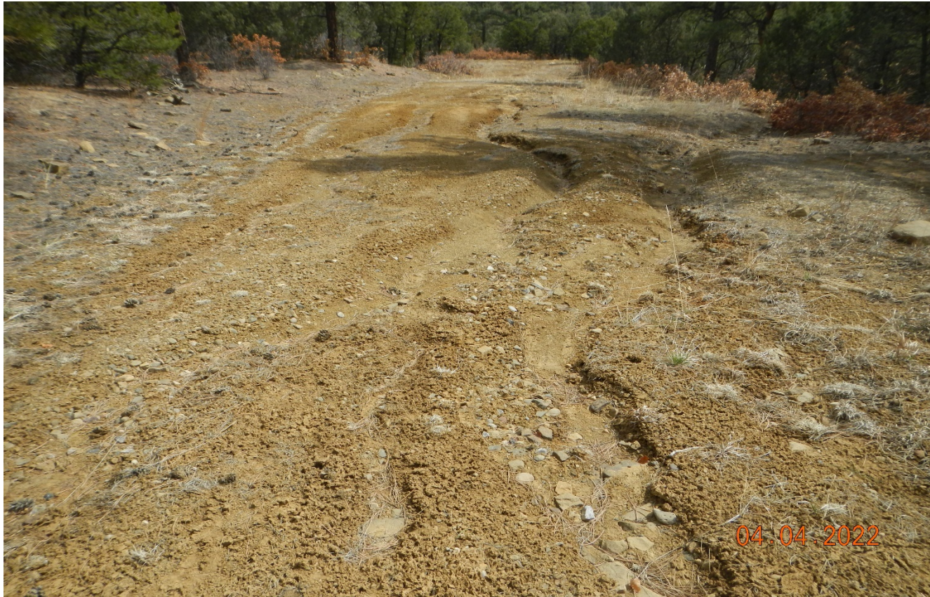
Photo 1. Facing east at the beginning of the access road. There is erosion channles along this area of the road that need to be repaired and stabilized.
