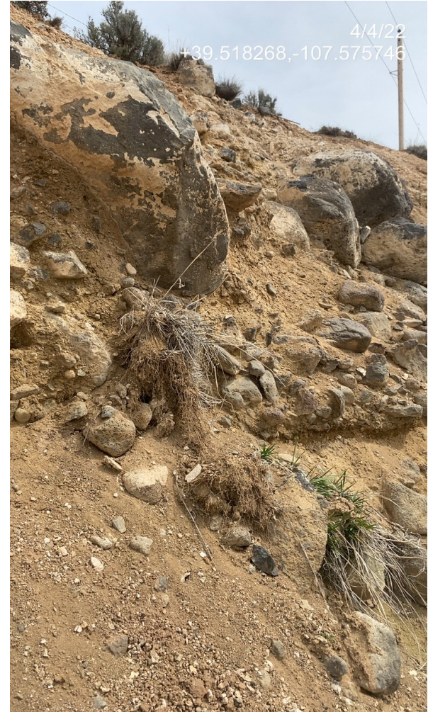
Photo 10. Photo taken from the center of the cut slope shows pedestalling and exposed roots on perennial vegetation colonizing the slope.
