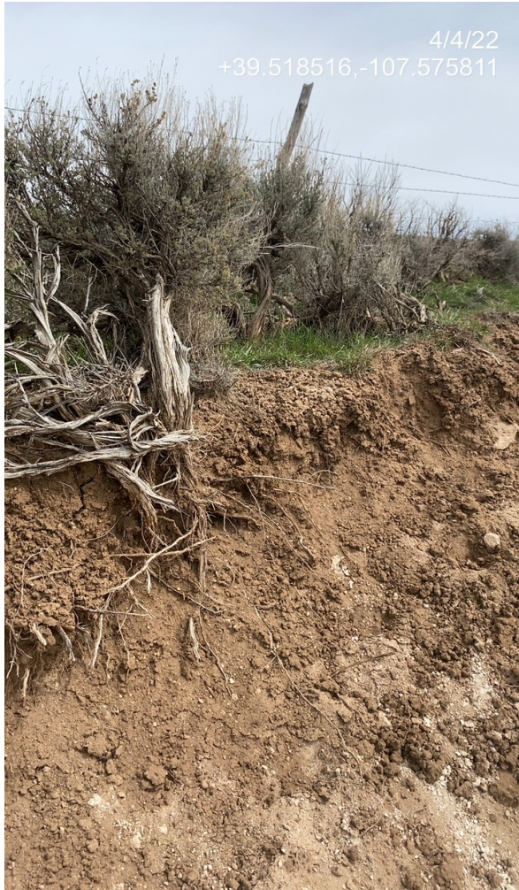
Photo 9. Photo taken from the top of the cut slope shows pedestalling and exposed roots on perennial vegetation adjacent to the Location.
