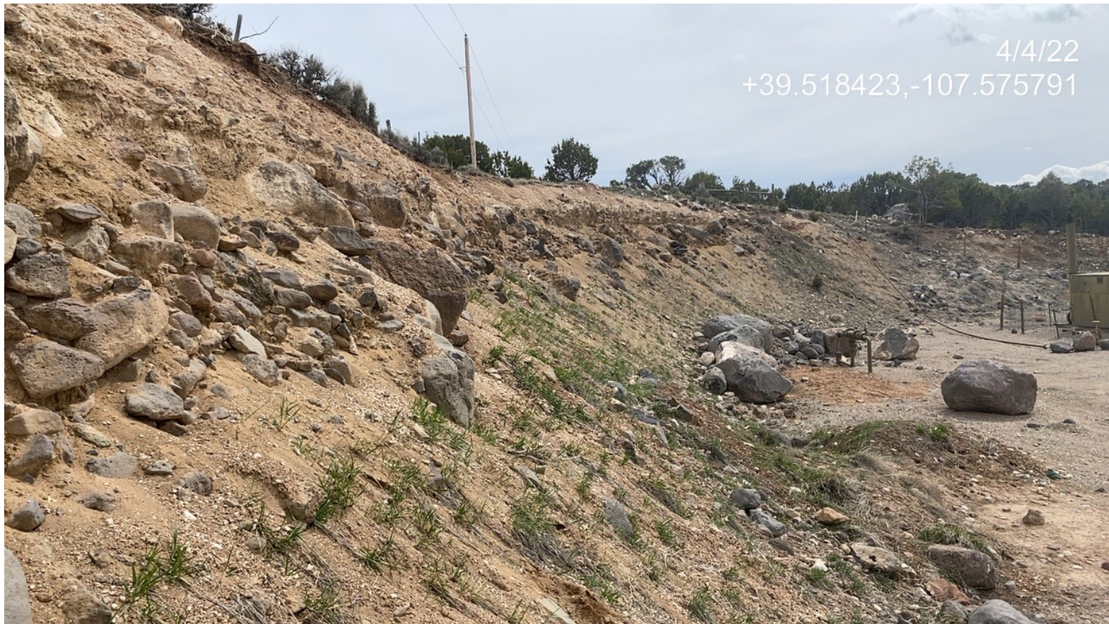
Photo 6. Photo taken from the east of the Location facing south shows an overview or the eroding cut slope.
