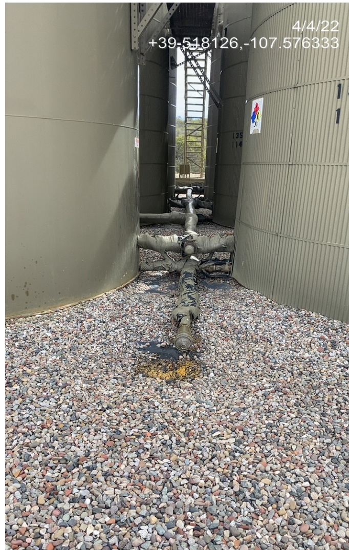
Photo 2. Photo taken from the tank battery shows staining below a valve.
