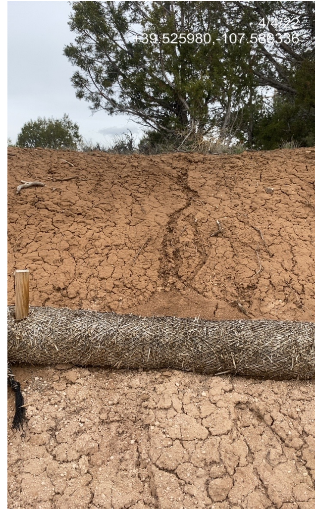
Photo 7. Photo taken from the east of the Location shows rill erosion occurring on the cut slope.
