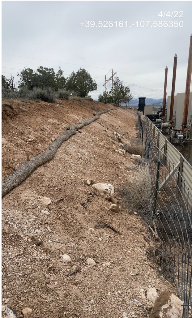
Photo 6. Photo taken from the east of the Location facing south shows an overview of the eroding cut slope.
