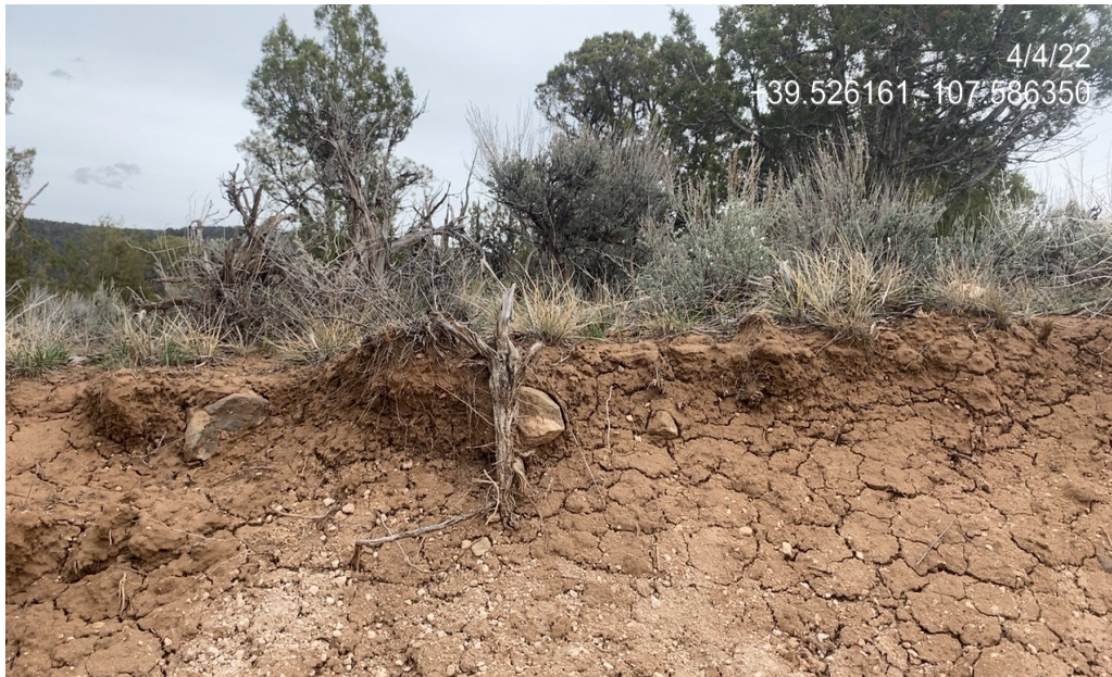
Photo 8. Photo taken from the east of the Location facing east shows undercutting and lateral erosion of cut slopes resulting in exposed roots and vegetation and soil loss from native plants communities off-Location.
