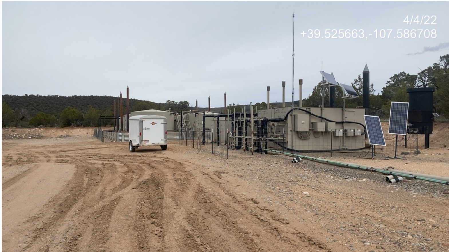
Photo 2. Photo taken from the southeast of the Location facing northeast shows storage of a trailer on Location. Photo also shows a lack of stabilization BMPs as is evidence by the presence of ruts.
