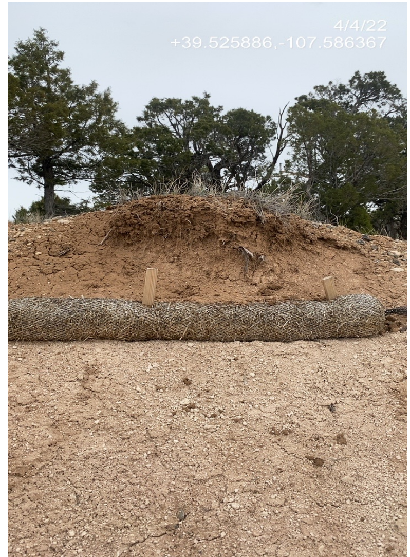
Photo 9. Refer to Photo 8 comment. A straw wattle does not appear to sufficiently prevent erosion.
