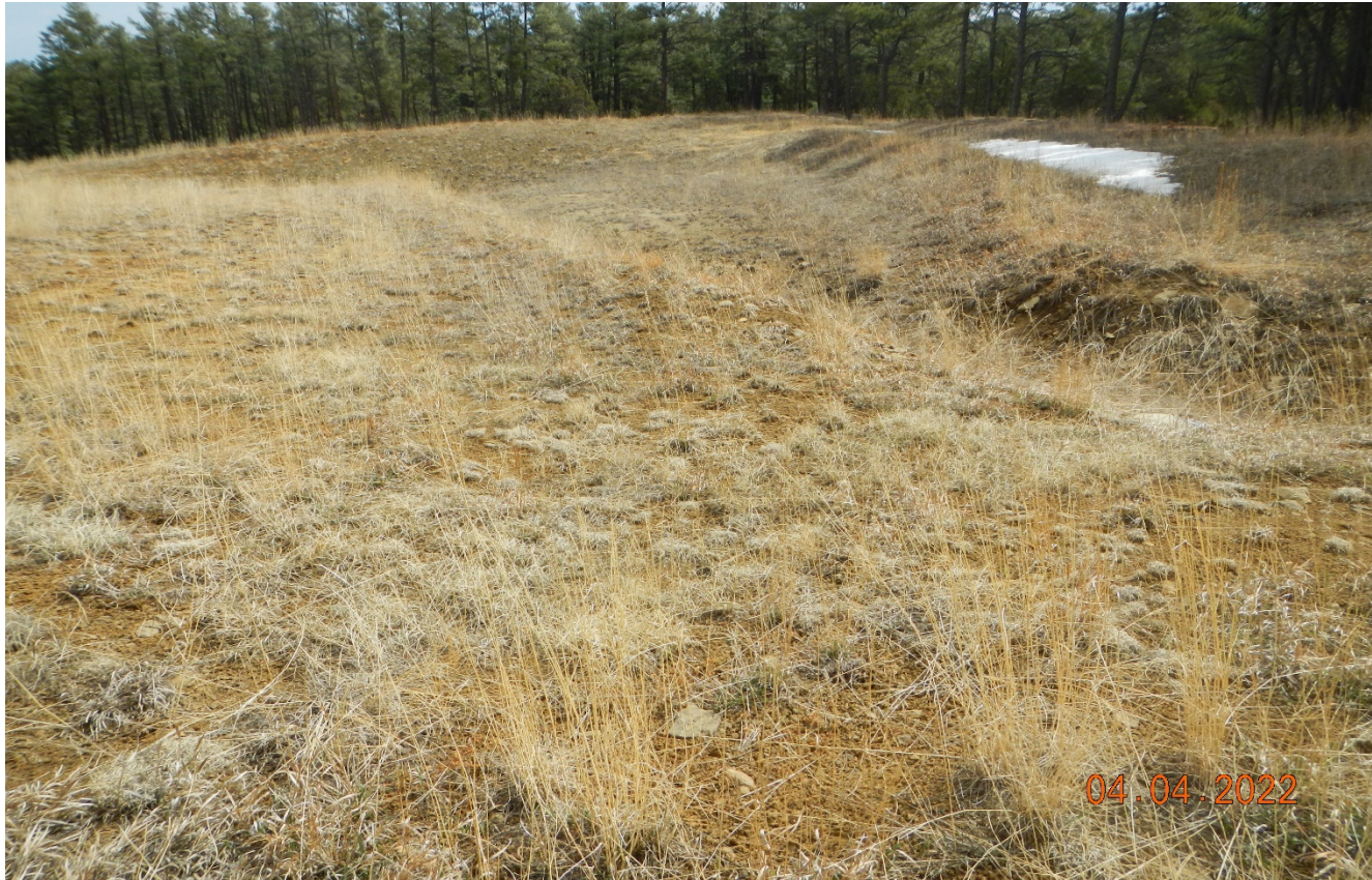
Photo 4. Facing east toward the cut slope which is stabilized.
