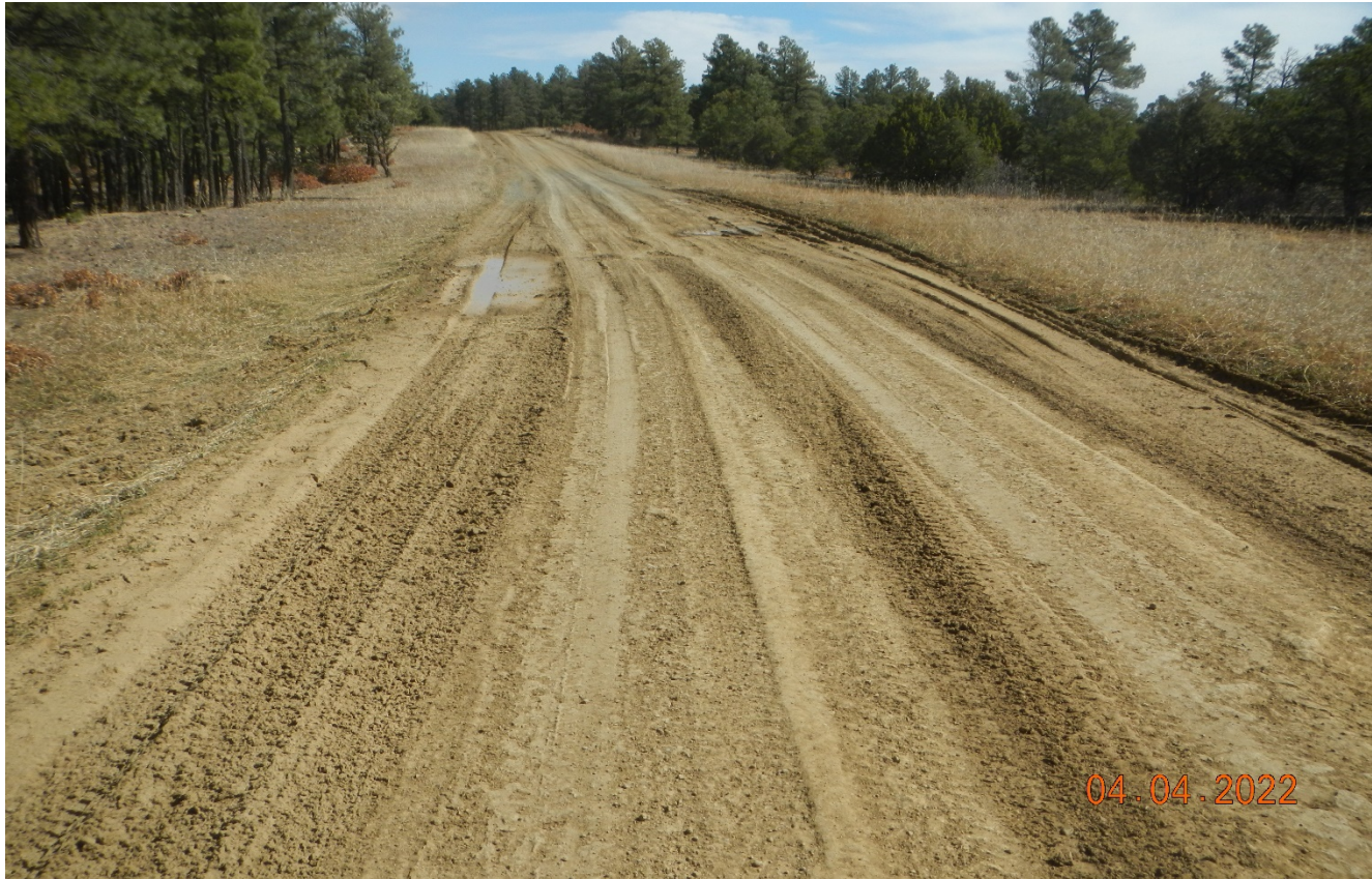
Photo 1. Facing north along the main road traveling to the location. There are areas of vehicle rutting. The road will need to be graded and maintained and areas may need additional stabilization.
