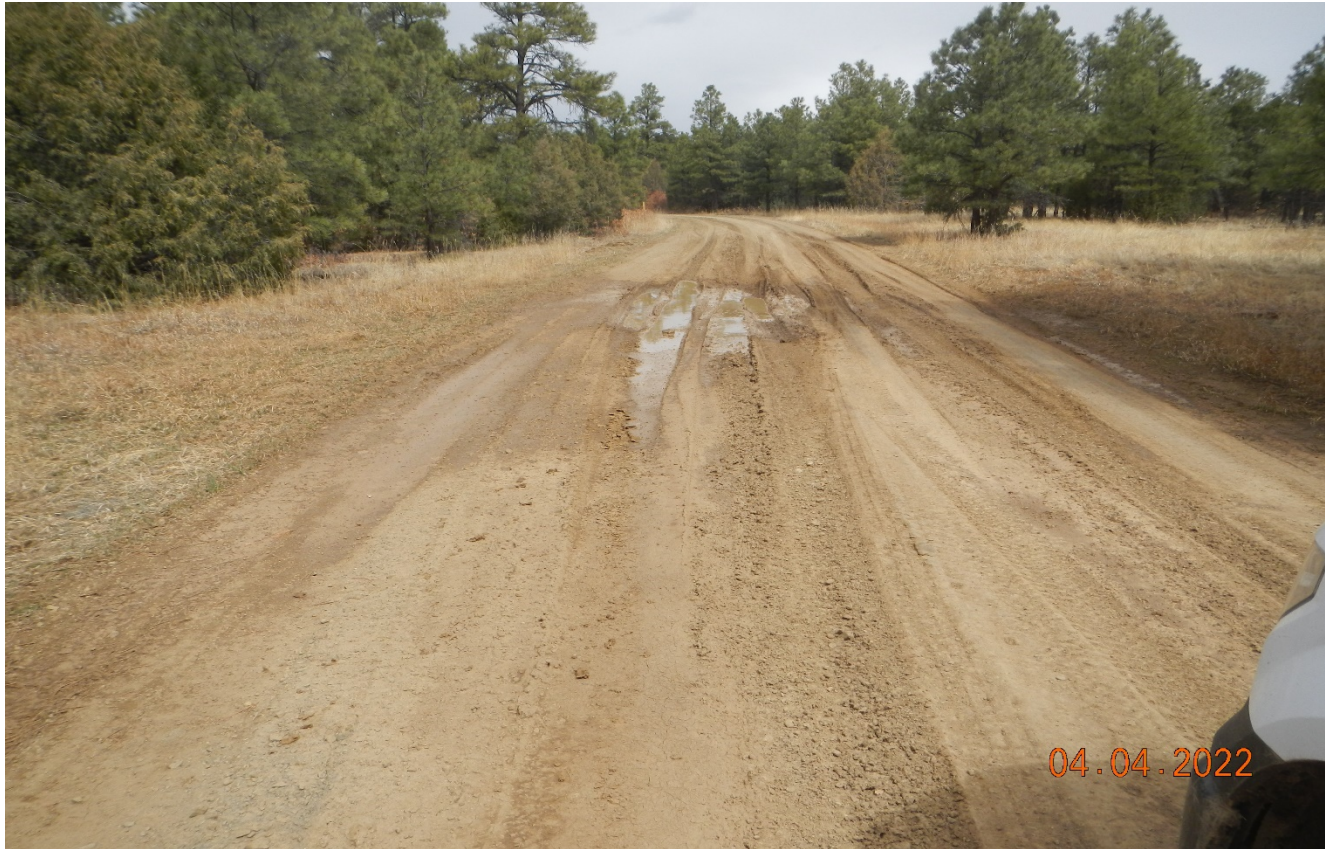
Photo 2. Facing northwest along the main road near the location. There are areas of vehicle rutting. The road will need to be graded and maintained and areas may need additional stabilization.
