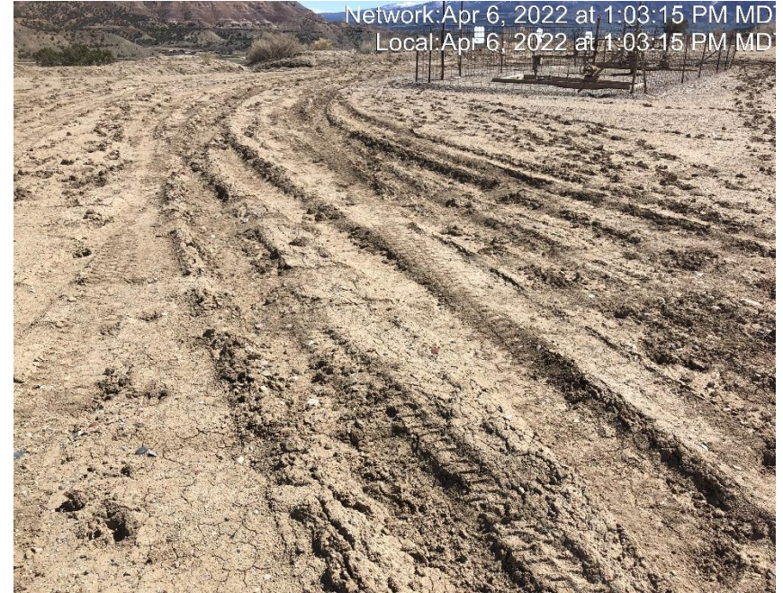
Photo #6376 Location lacks stabilization.
