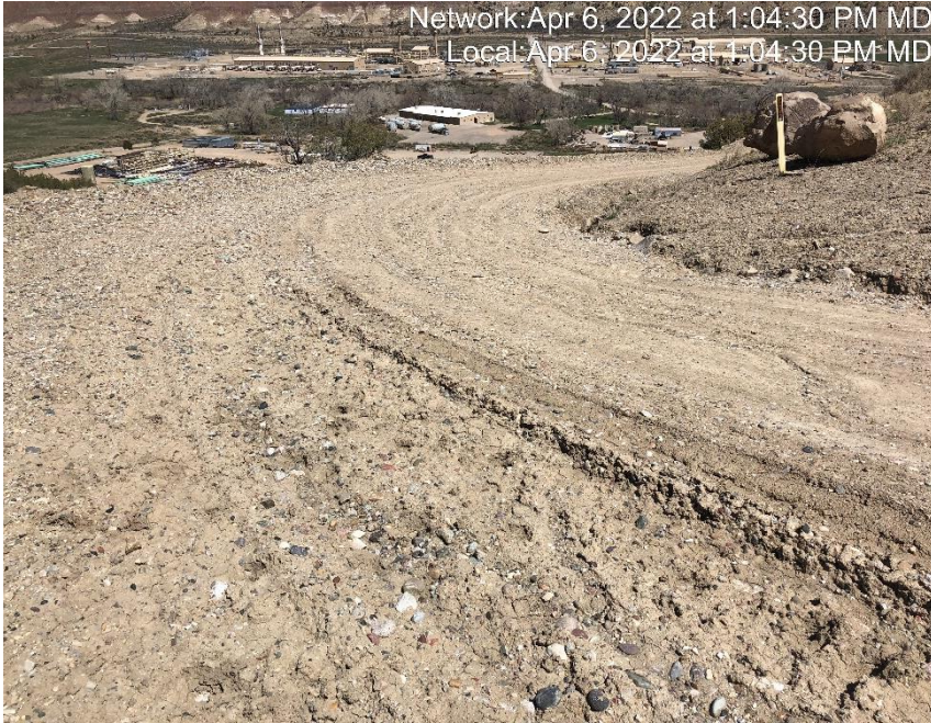
Photo #6379 Insufficient tracking control at entrance to location
