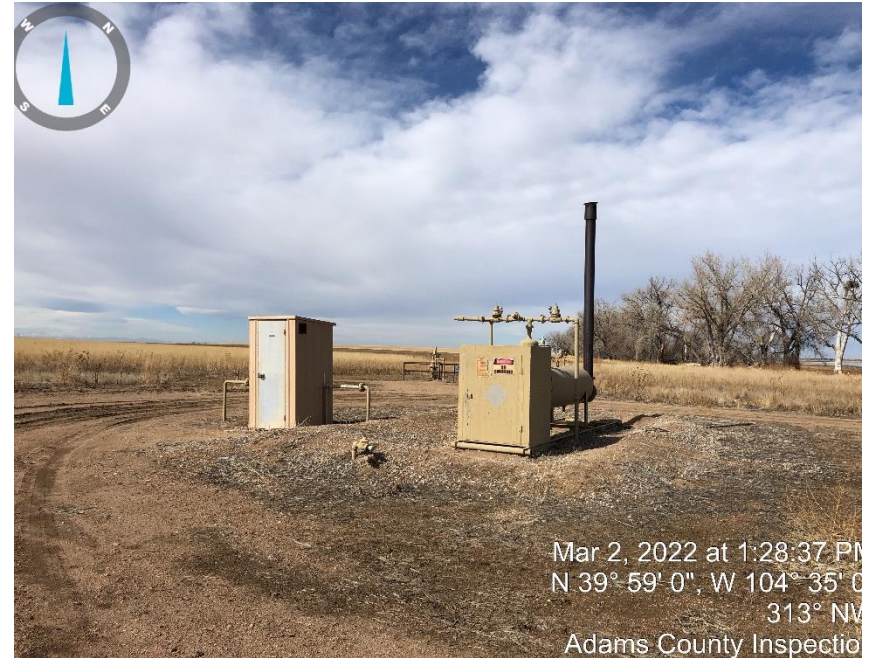
Photo #2 Meter and Separator.
