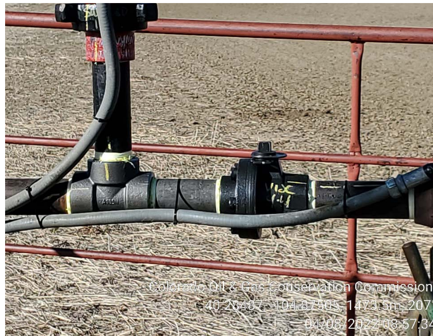
Valve leak on 4/8/2022
