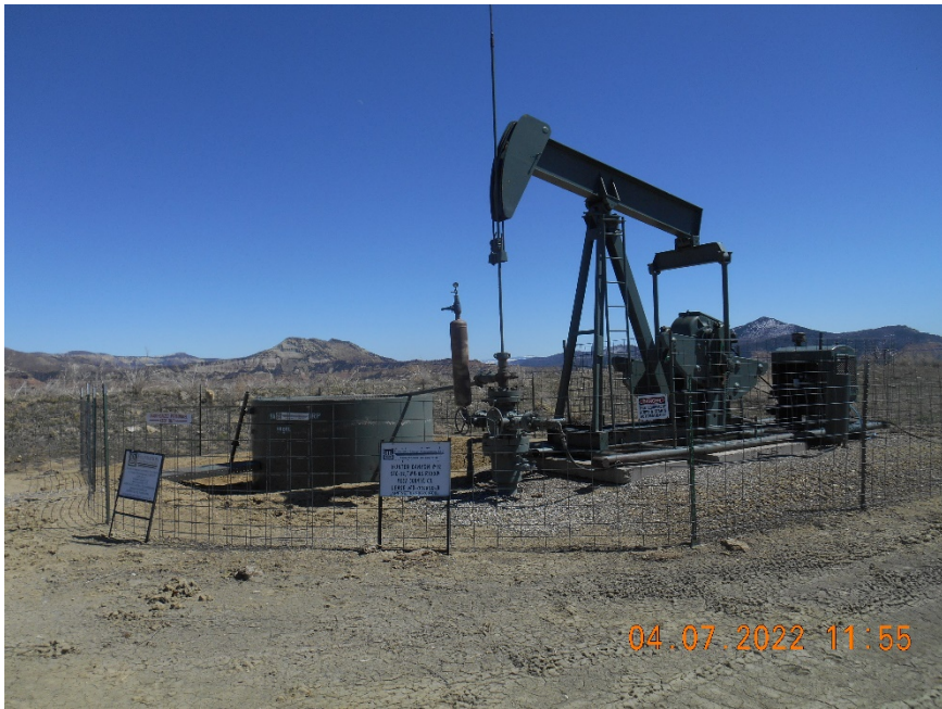
Wellhead with Pump jack, fence and sign
