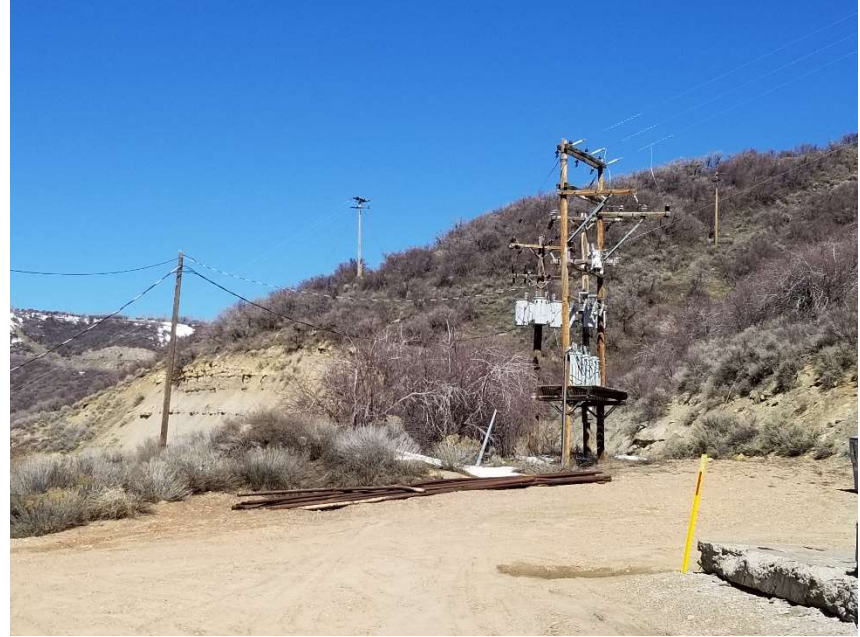
Photo 2. Tubing stored on location.
