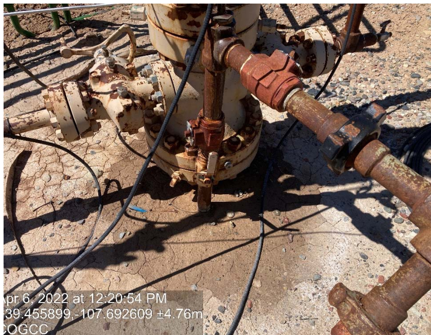
Leaking Braden head line
