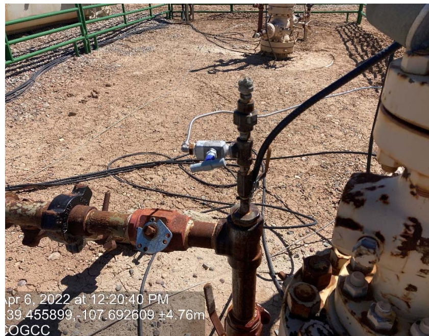
Leaking Braden head line
