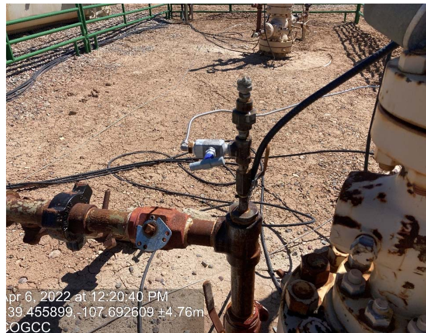
Leaking Braden head line
