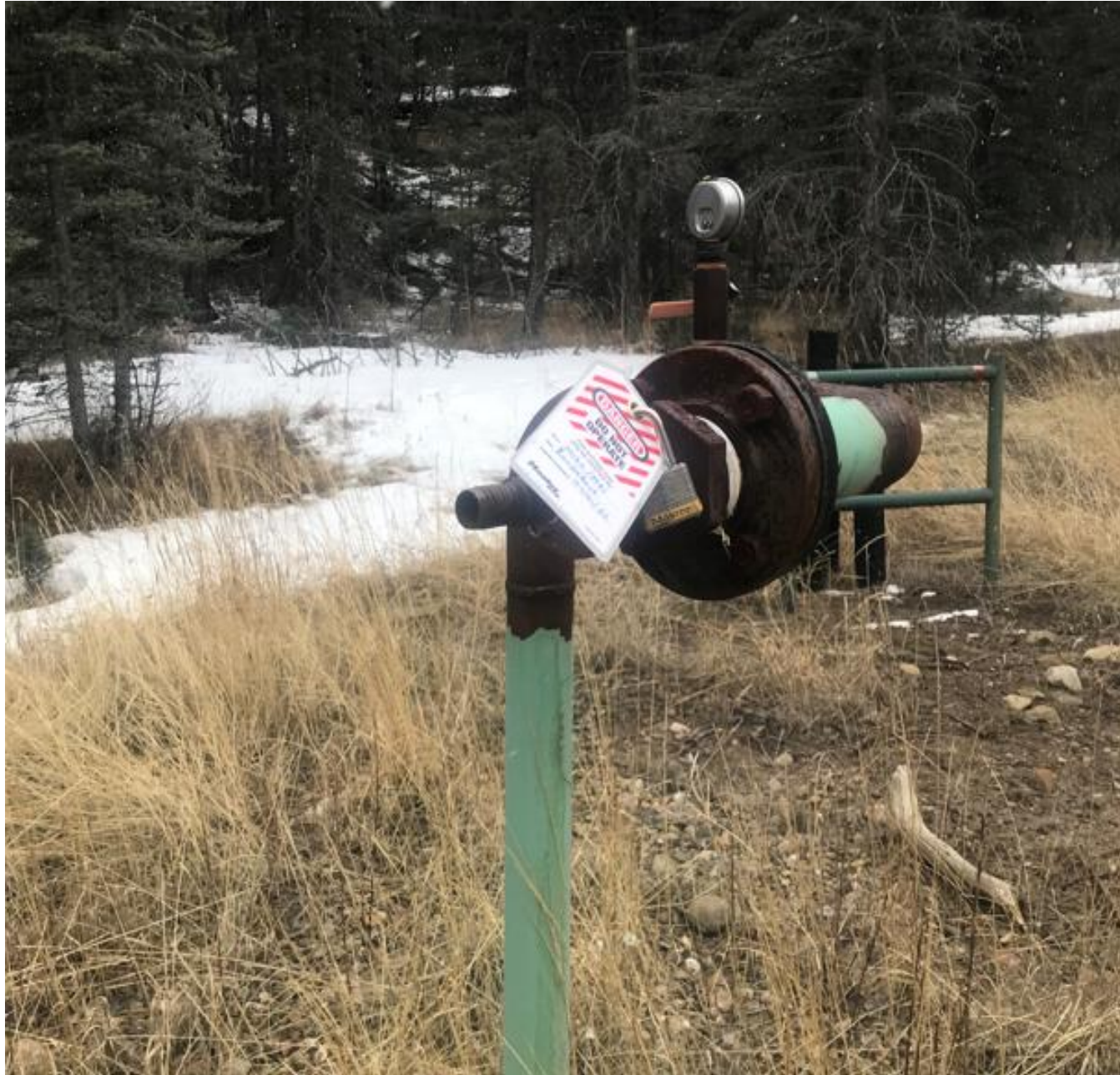
PHOTO 3: THE GAS LINE HAS BEEN LOCKED OUT AND APPROPRIATELY LABELED WITH LO/TO TO COMPLY WITH RULE 606. CORRECTIVE ACTION COMPLETED 04/01/2022.
