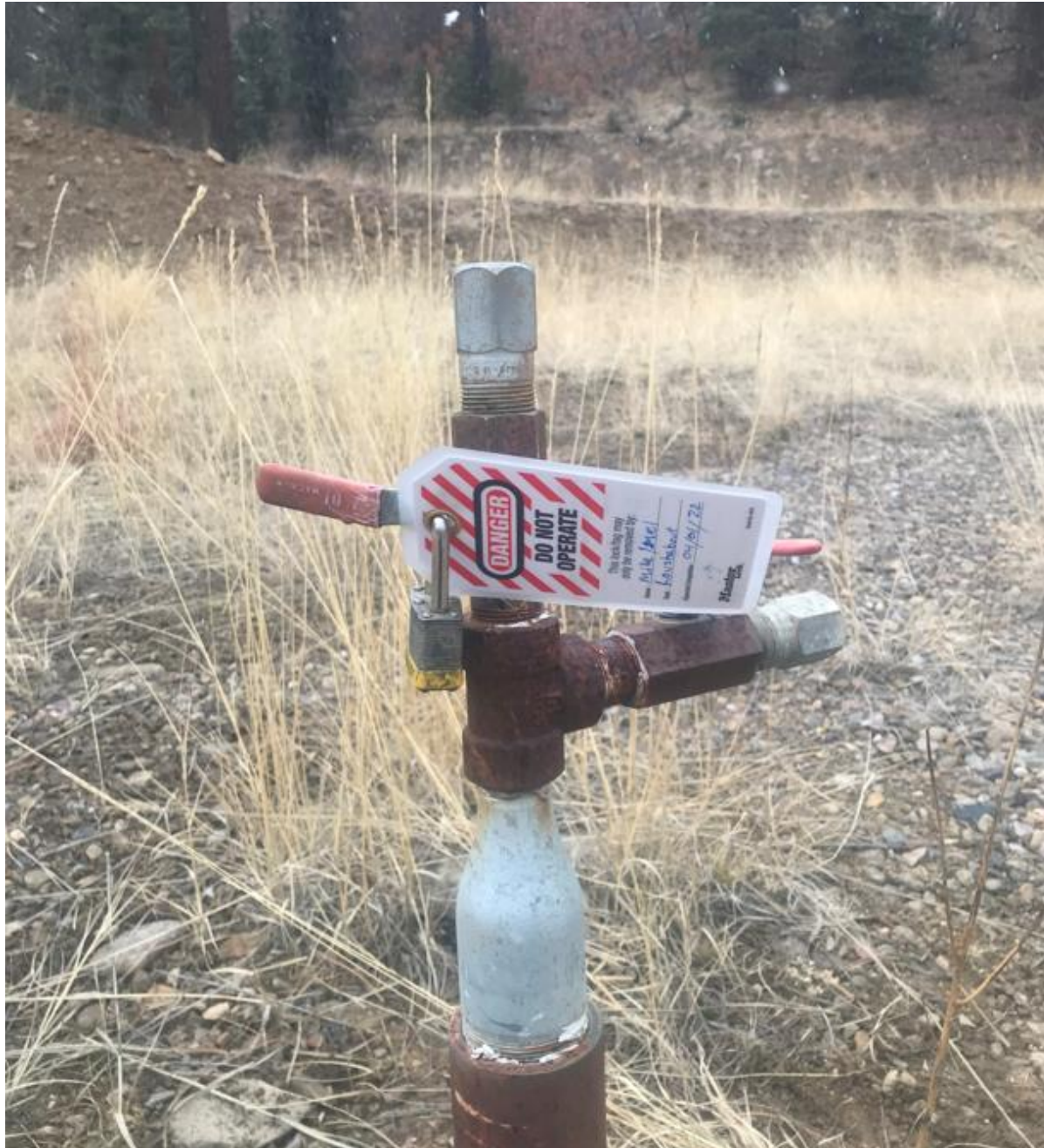
PHOTO 1: THE 1" RISER HAS BEEN LOCKED OUT AND APPROPRIATELY LABELED WITH LO/TO TO COMPLY WITH RULE 606. CORRECTIVE ACTION COMPLETED 04/01/2022.
