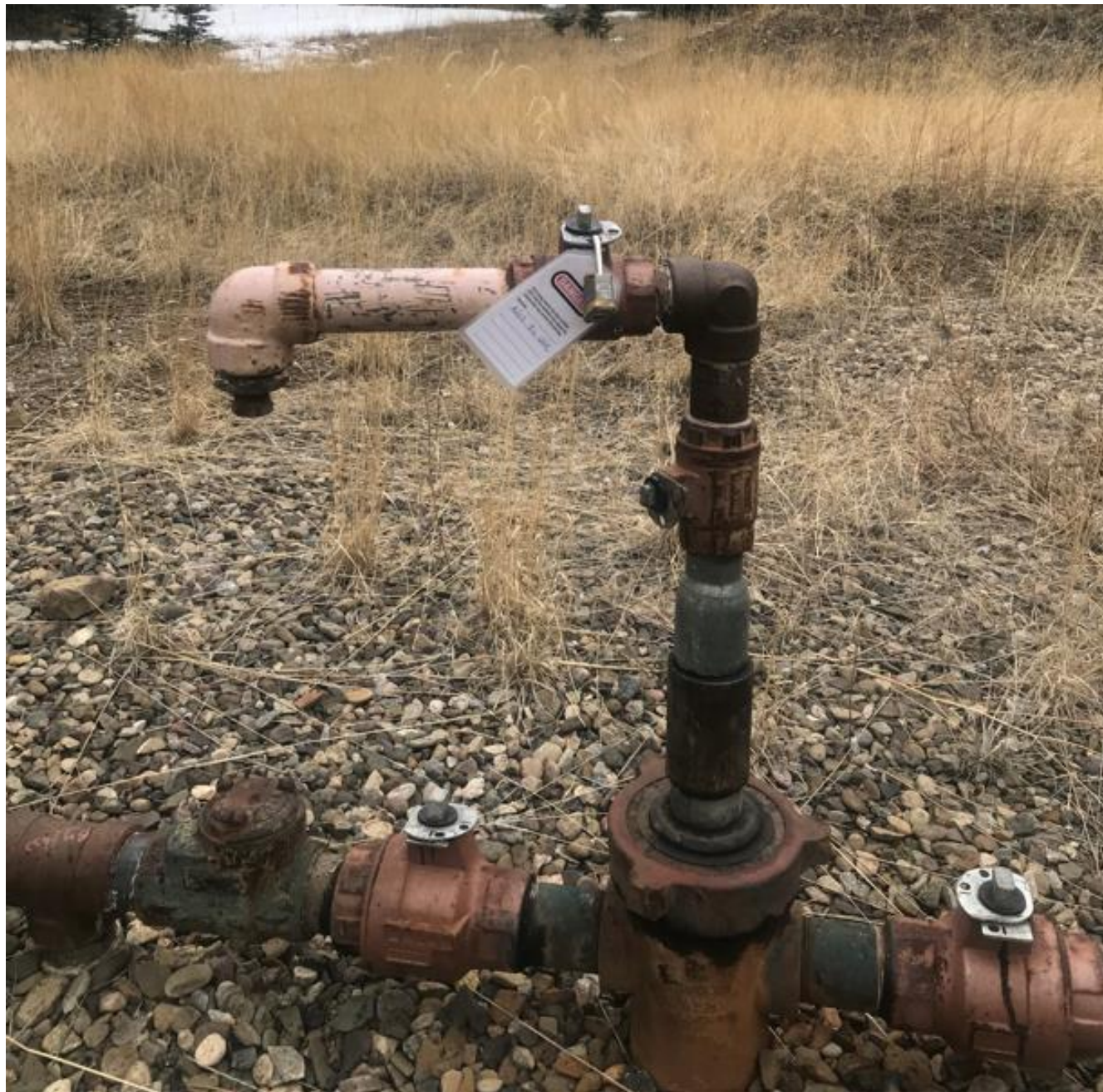
PHOTO 2: THE WELLHEAD HAS BEEN LOCKED OUT AND APPROPRIATELY LABELED WITH LO/TO TO COMPLY WITH RULE 606. CORRECTIVE ACTION COMPLETED 04/01/2022.
