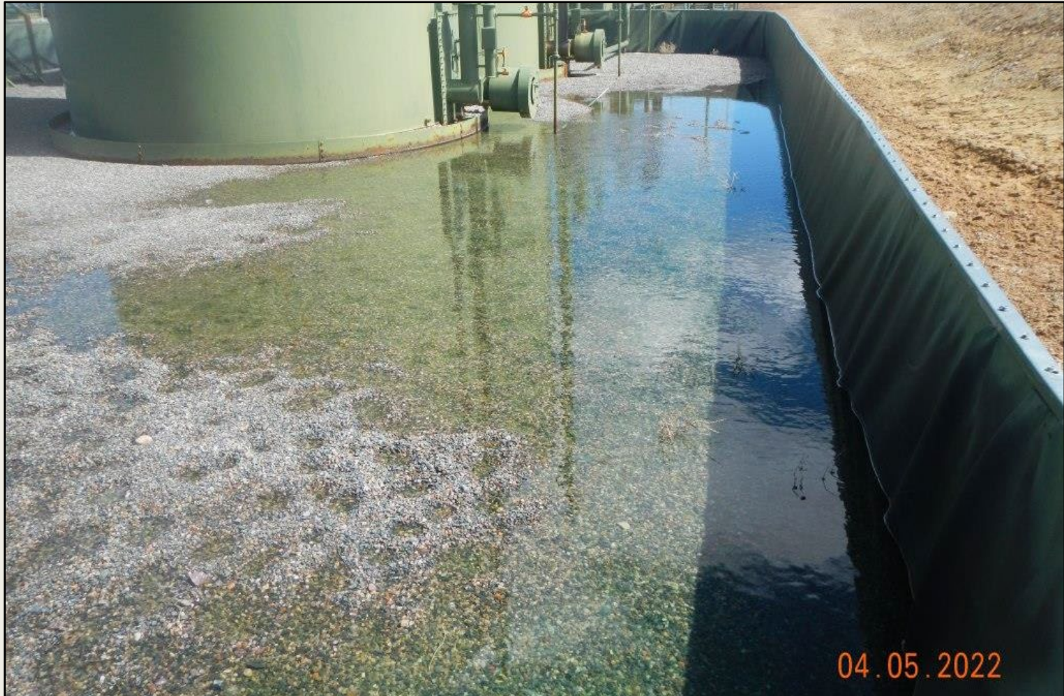
Photo 3. View of water ponding within secondary containment. It appears ponding may be result of long-term slow leak from tank plumbing.
