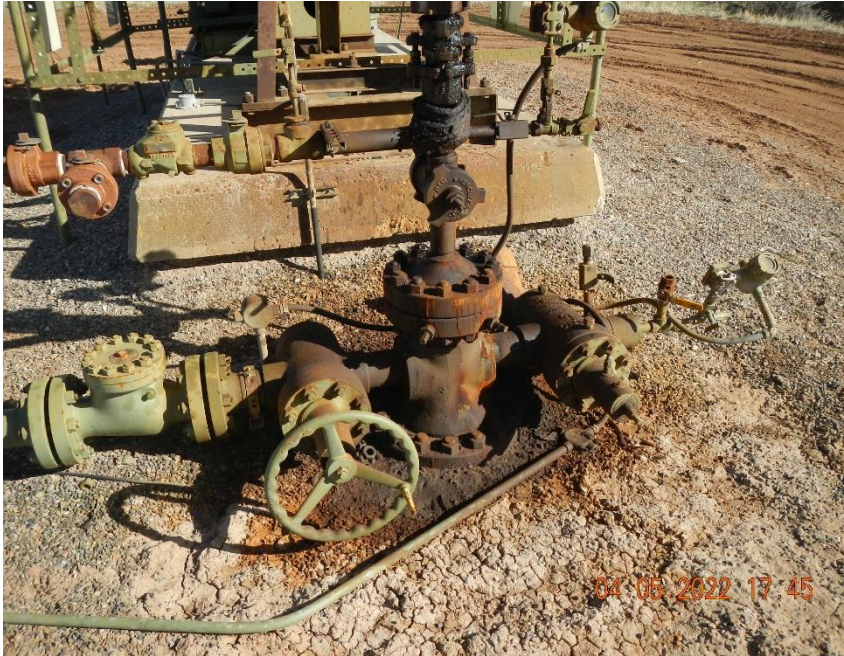
Well head and surrounding area are stained and wet.
