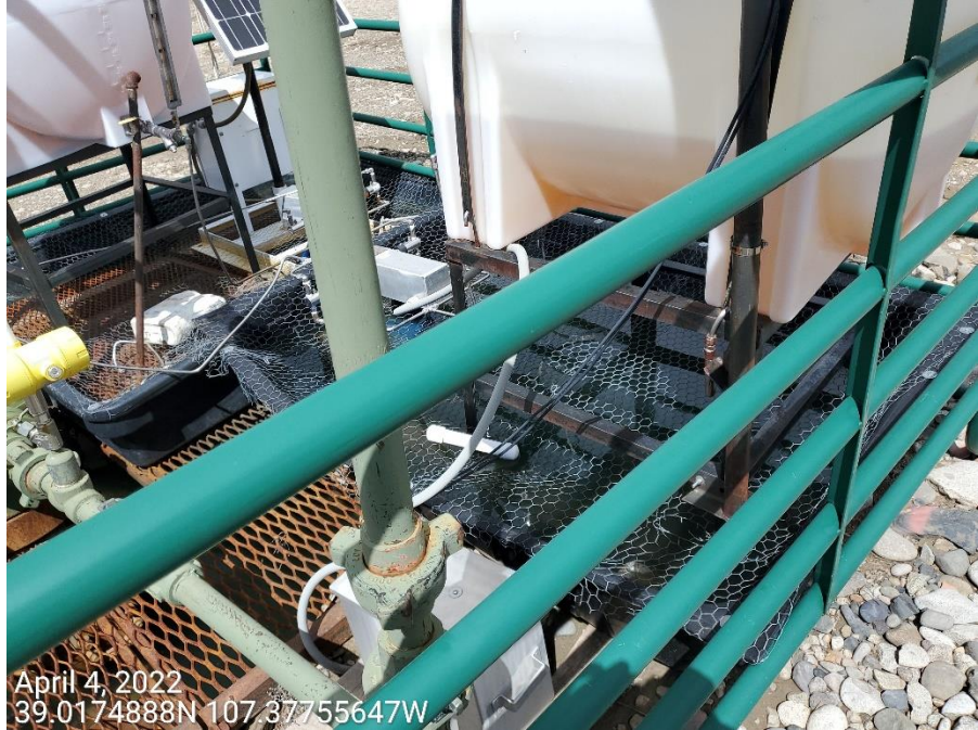
Photo 3: Photos example showing secondary containment for tanks adjacent to the wells have filled with fluids, and are no longer adequate to contain a spill.
