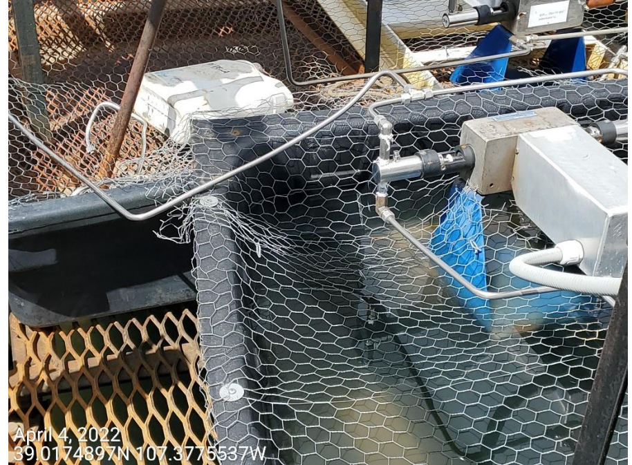
Photo 3: Photos example showing secondary containment for tanks adjacent to the wells have filled with fluids, and are no longer adequate to contain a spill.
