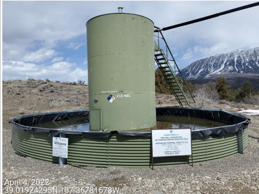
Photo 6: Signage at tank battery remains inadequate; sign missing information per Rule 605.e.. EMS# or 911, Nearest public road, and API. First letter of tank contents on side of the tank remains missing.
