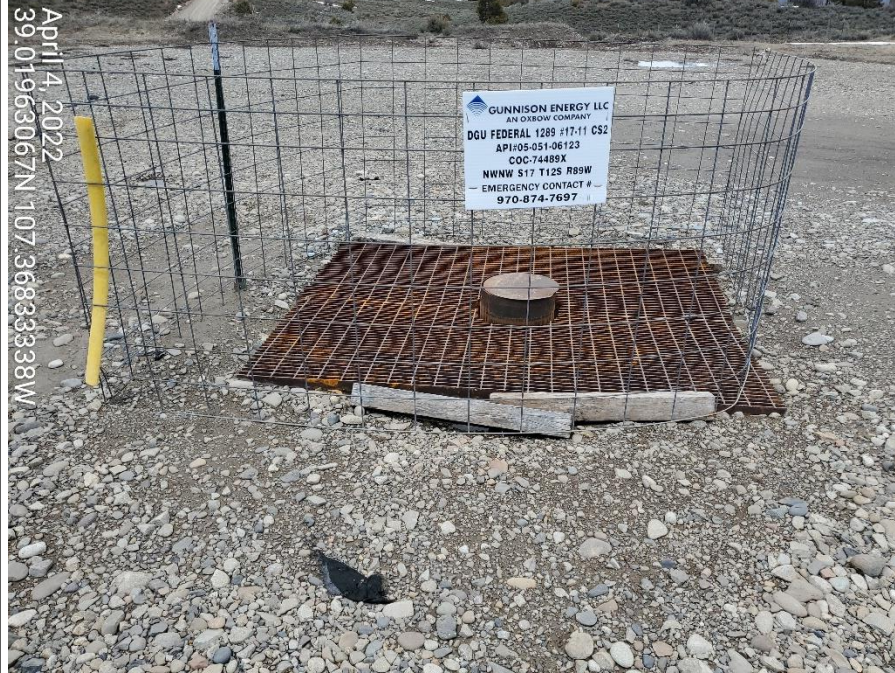
Photo 5: Photos show conductor and cellar for Well API #051-06213; records show well is abandoned; conductor and cellar for this well have not been plugged and reclaimed per Rule 406 requirements; conductor and cellar remaining; plate on top of the conductor pipe not welded per requirements. No Form 4 - "Report of work done" to report plugging of the conductor has been submitted. Well conductor requires plugging and reclamation.
