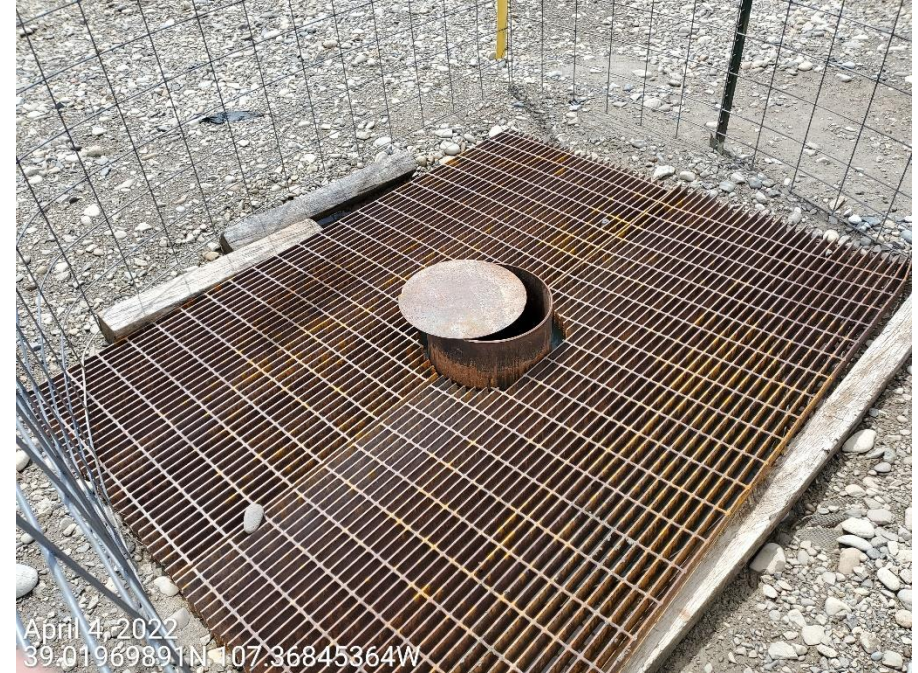
Photo 5: Photos show conductor and cellar for Well API #051-06213; records show well is abandoned; conductor and cellar for this well have not been plugged and reclaimed per Rule 406 requirements; conductor and cellar remaining; plate on top of the conductor pipe not welded per requirements. No Form 4 - "Report of work done" to report plugging of the conductor has been submitted. Well conductor requires plugging and reclamation.
