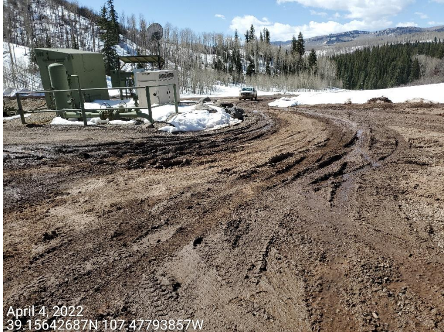
Photo 3: Photos show inadequate stabilization and tracking BMPs on the Location.
