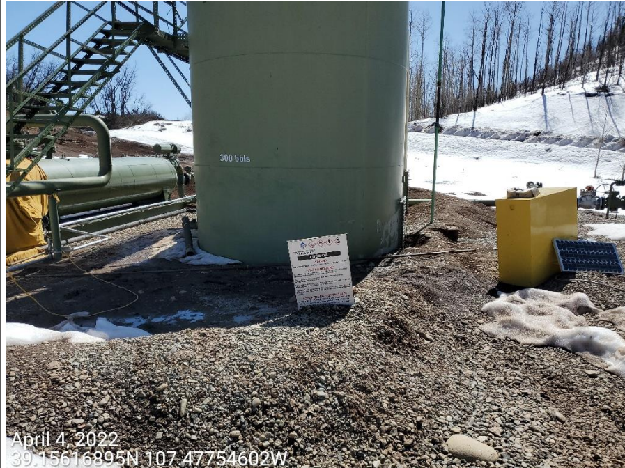
Photo 4: Photos show adequate, impervious containment has not been installed at the tanks in accordance with good engineering practices.
