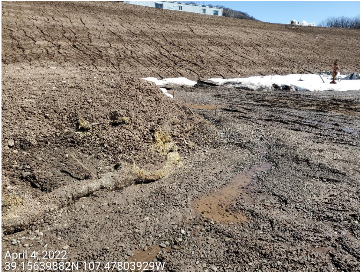
Photo 2: Photos taken from the soil stockpile on the Location; Operator has placed a straw wattle at base of stockpile; BMP has not been installed per good engineering practices, or maintained in a proper functioning condition. BMPs at stockpile remain inadequate.
