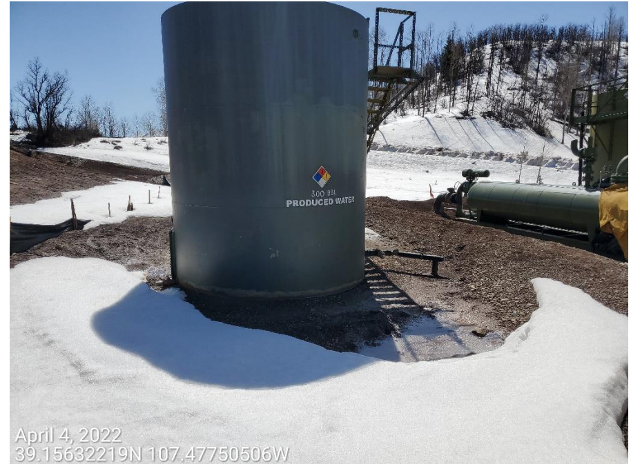
Photo 5: Photos show adequate, impervious containment has not been installed at the tanks in accordance with good engineering practices.
