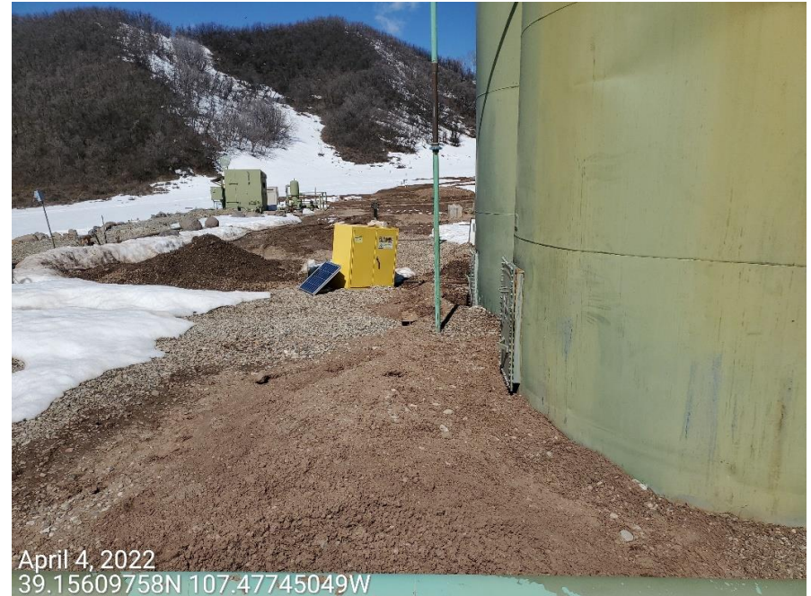
Photo 4: Photos show adequate, impervious containment has not been installed at the tanks in accordance with good engineering practices.
