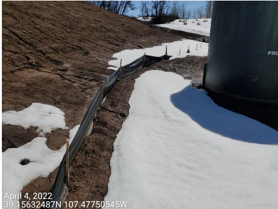
Photo 5: Photos show adequate, impervious containment has not been installed at the tanks in accordance with good engineering practices.
