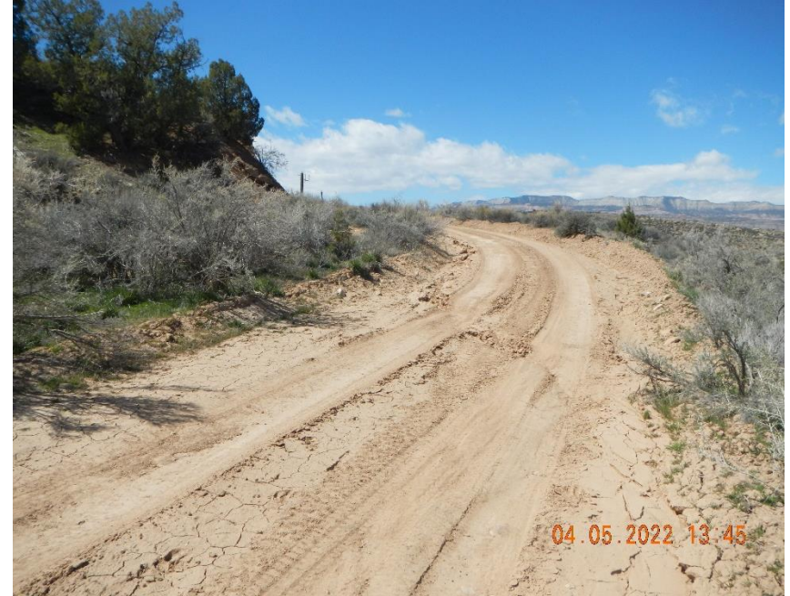
Storm water rills crossing roadway.
