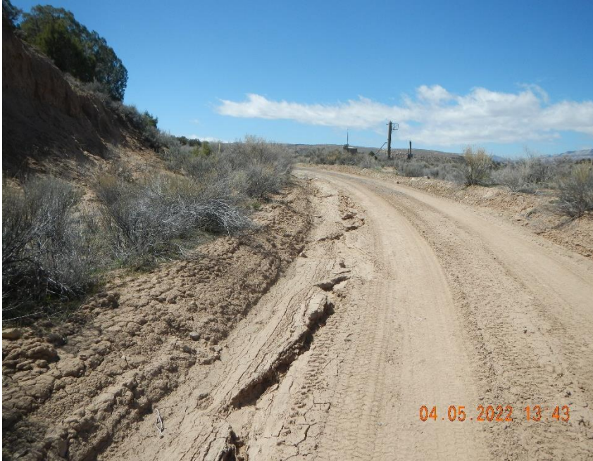
Road ditches are washing and sediment moving.
