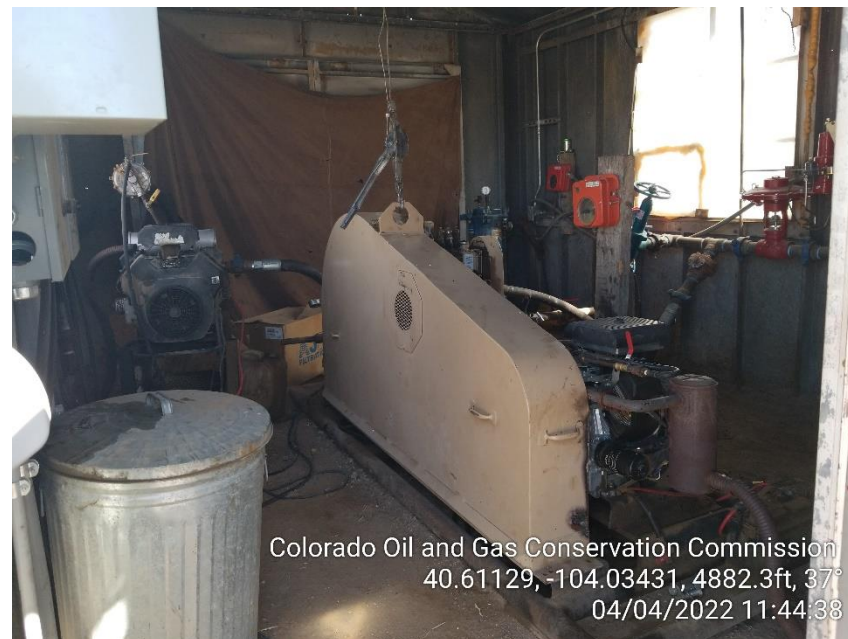
Photo 6 – Injection Pump
