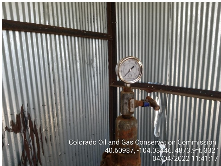
Photo 3 – Tubing Gauge
