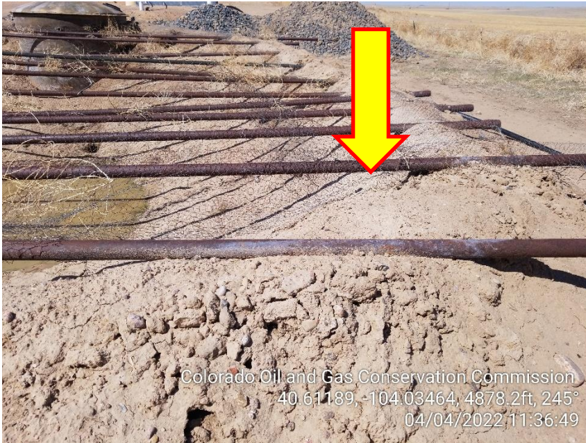
Photo 7 – Hole/Gap in Pit Netting
