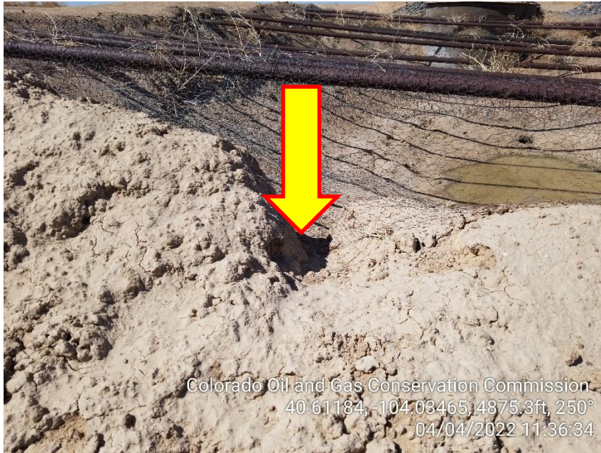
Photo 5 – Hole/Gap in Pit Netting
