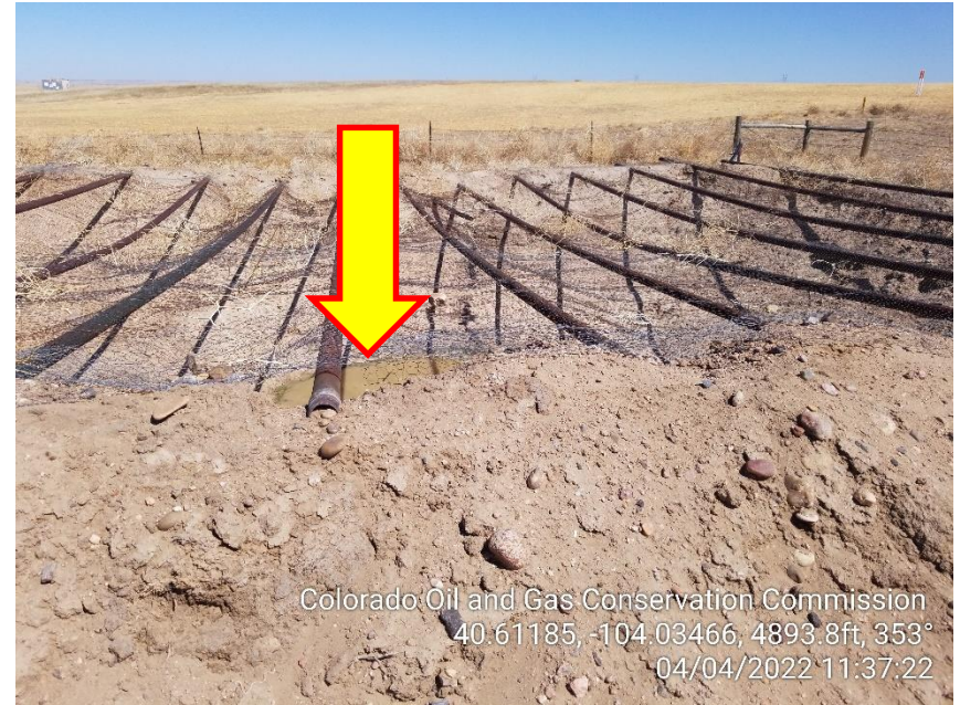
Photo 8 – Hole/Gap in Pit Netting
