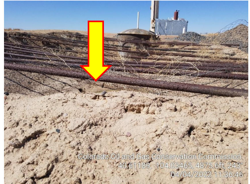
Photo 6 – Hole/Gap in Pit Netting
