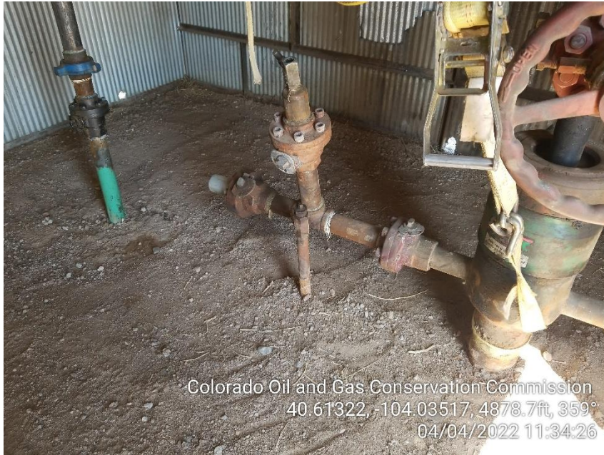
Photo 5 – Bradenhead/Surface Casing
