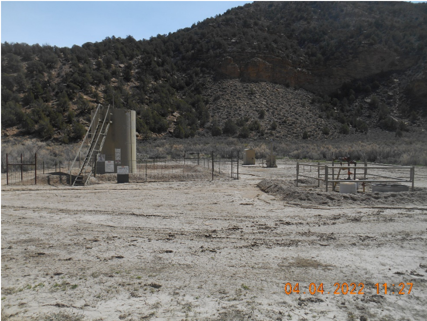
Location overview looking E.
