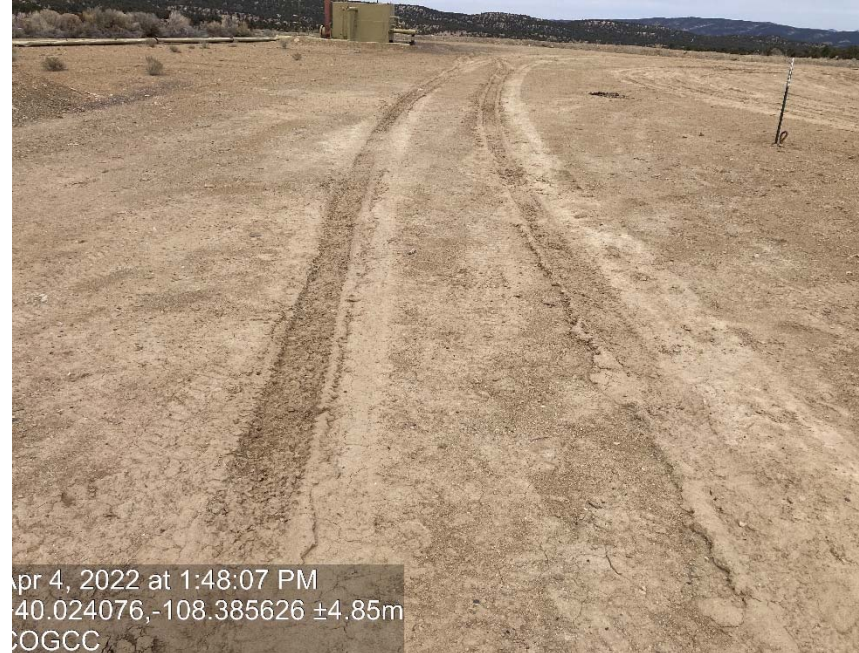
Lack of stabilization/compaction
