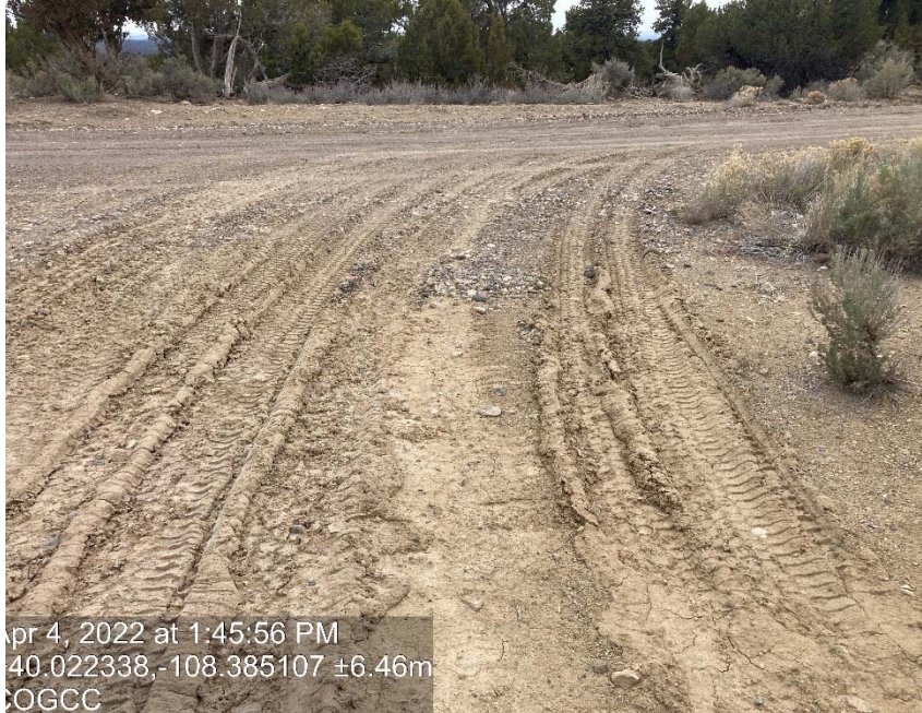
Lack of stabilization/compaction
