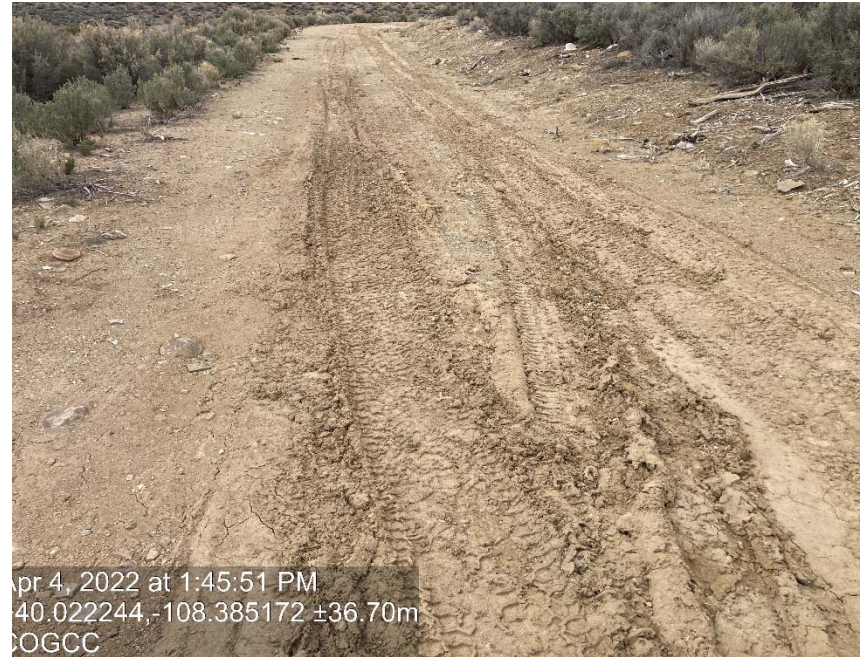
Lack of stabilization/compaction
