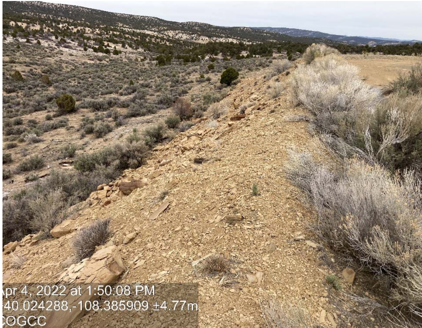
Lack of stabilization/compaction/erosion
